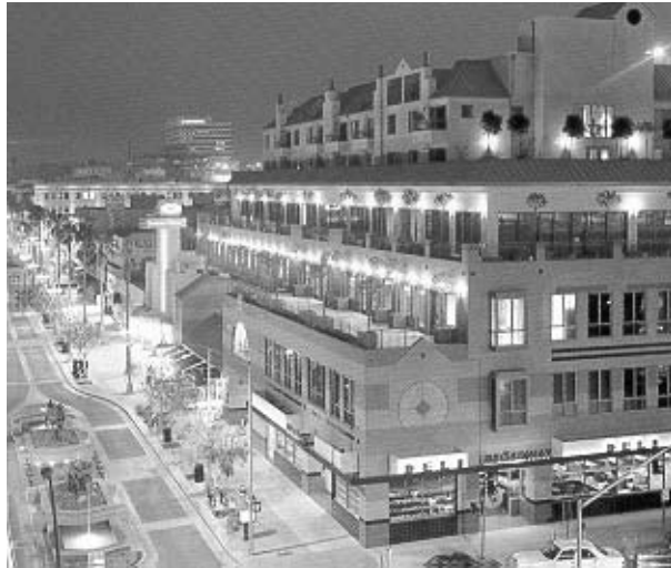
Building setbacks (BSM-3) such as those seen on this building in Santa Monica, CA can be utilized to maintain a pedestrian scale to the street and to provide outdoor space to upper floor users.
