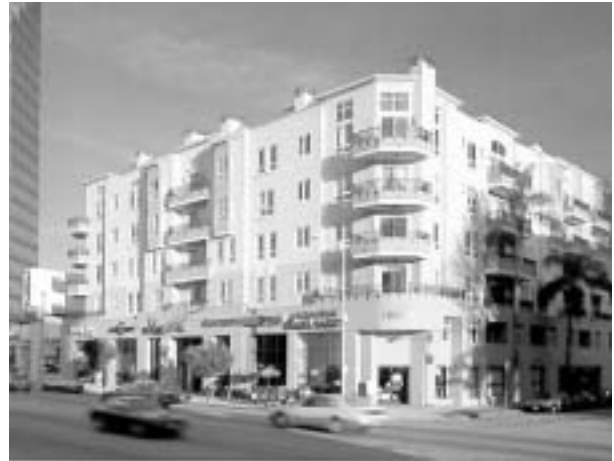
Generally, signs should not extend above the window sills of the second floor (S-2).
