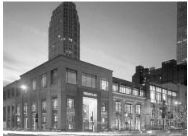
Upper floor facades should consist of at least 25% window space (F-1) as shown on this building in Chicago, IL.
