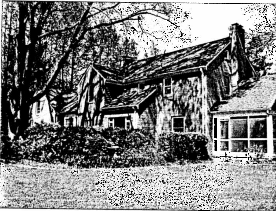
9200 Darnestown Road View of south (rear) elevation from southeast
