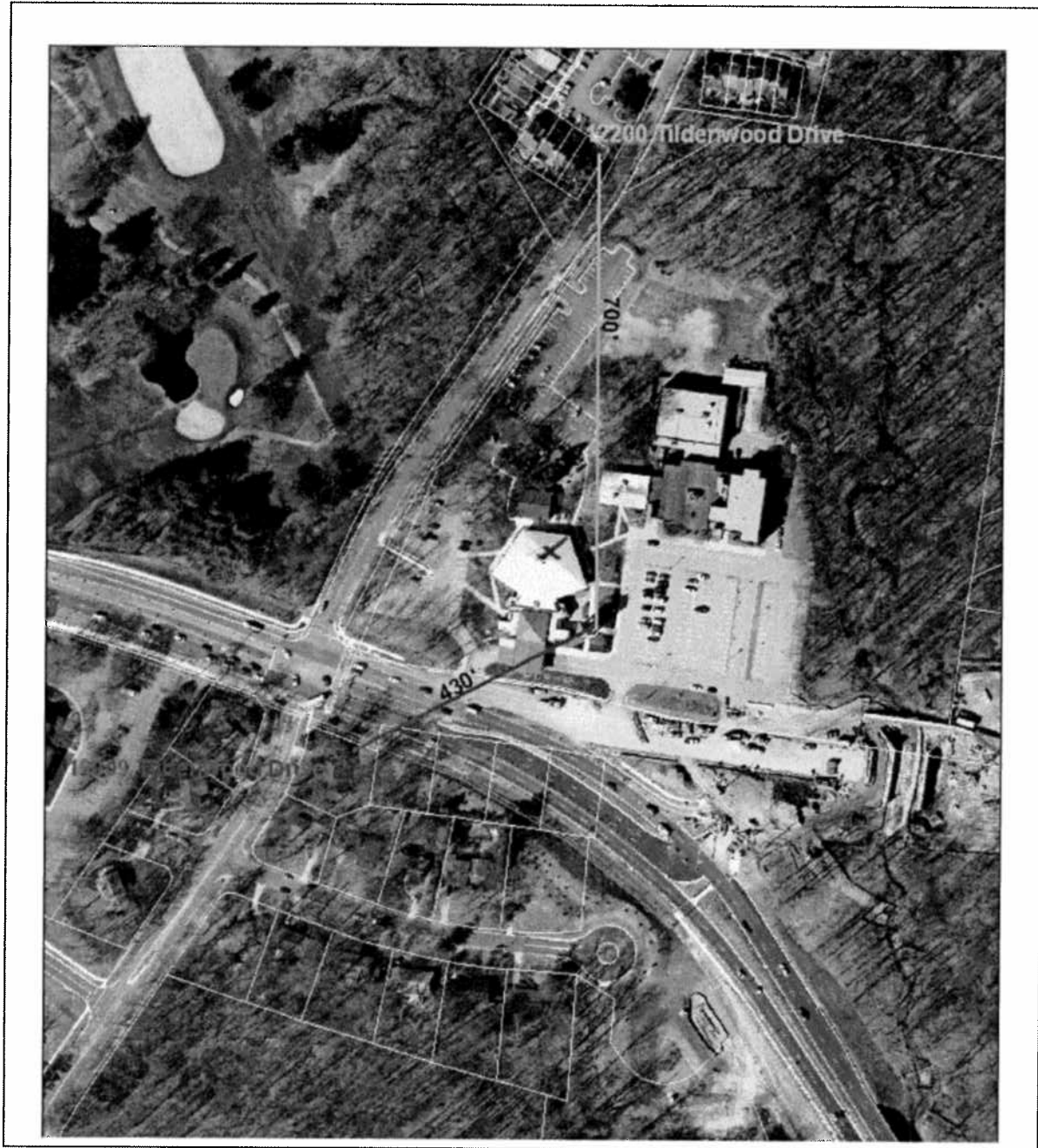
Aerial Photograph of Site and Abutting Properties
