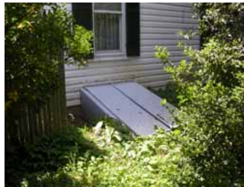
East Elevation, basement doors
