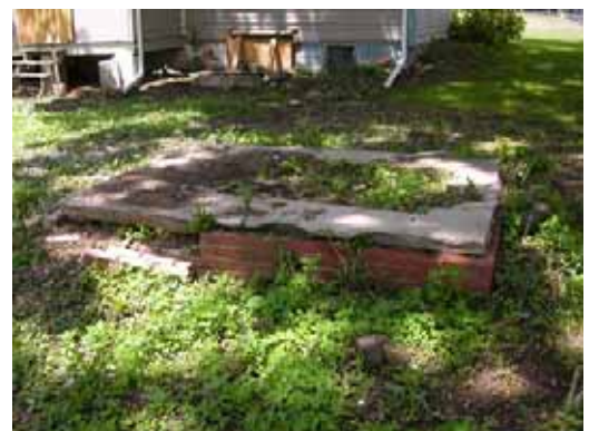
Foundation at southeast corner of property
