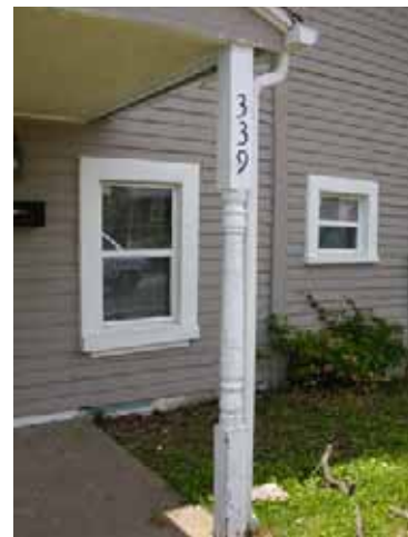
North Façade Column detail
