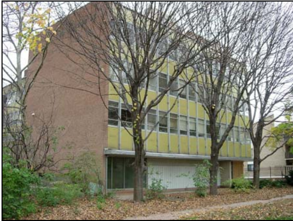
South (front) facade 2004- Peerless Rockville
