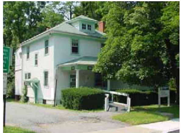
150 Maryland Avenue, West facade
