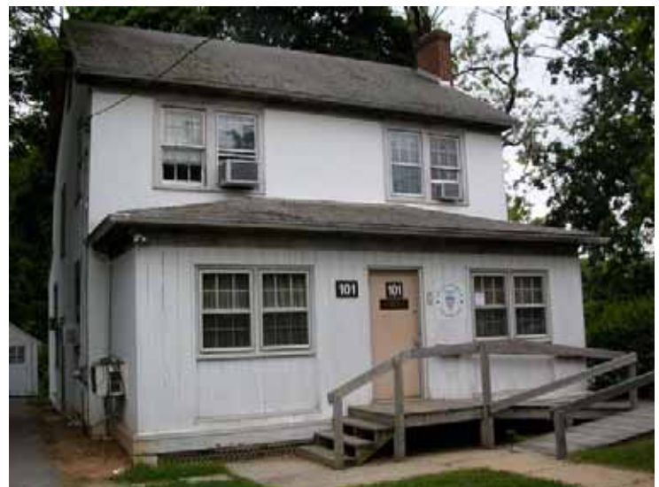
101 Fleet Street, North façade
