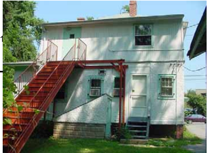
150 Maryland Ave, East façade
