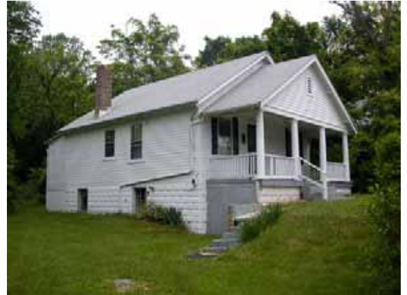
213 Monroe Street, South East Facades
