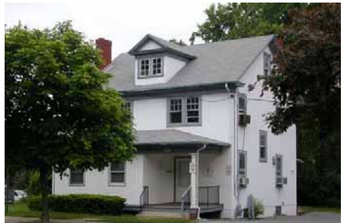
105 Fleet Street, North façade
