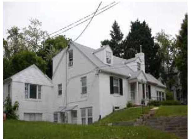
209 Monroe Street, South and East (front) Facades
