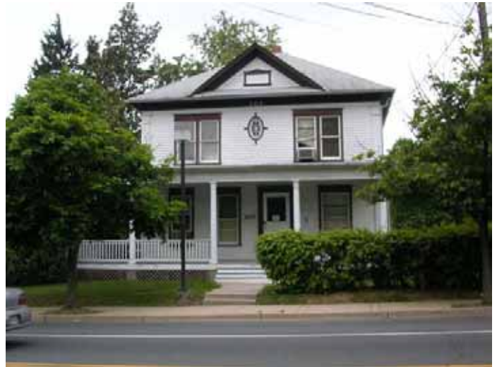
107 Fleet Street, North (front) façade
