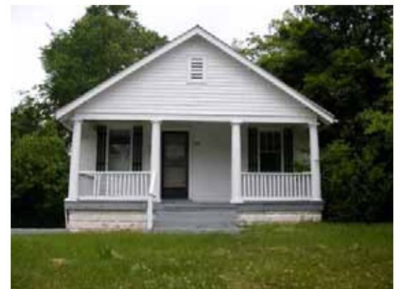
215 Monroe Street, East Facade
