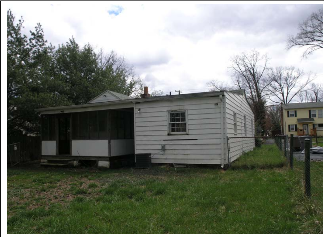
N & W Elevations, Rear and left side
