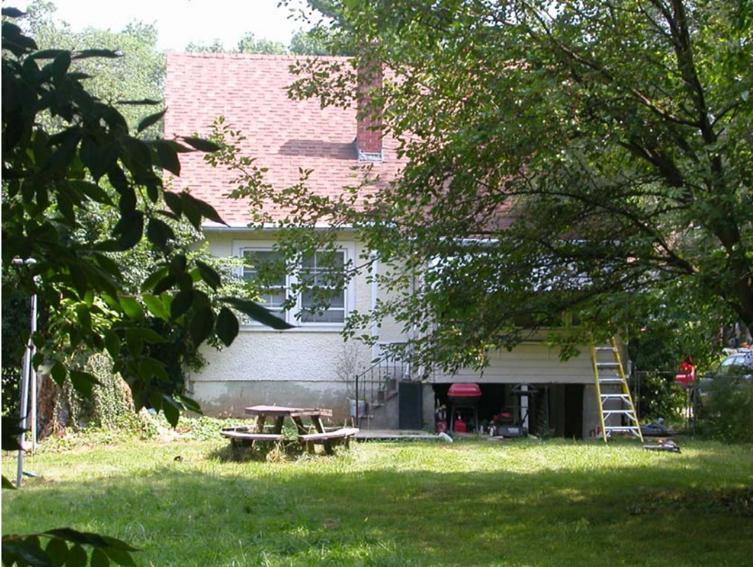
View of south elevation from alley
