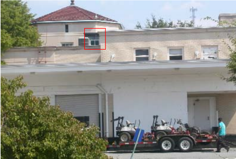
Rear elevation, taken from west boundary line of Burbanks. View of roof monitor outlined in red square.
