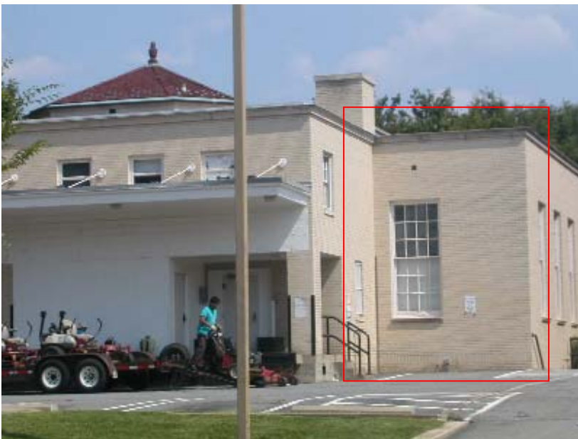
Rear elevation, southwest corner where elevator tower is to be located
