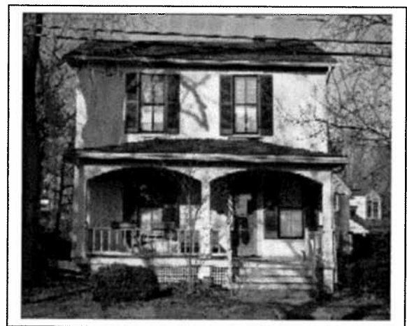
108 N. Adams, Façade (east elevation)
