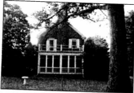
East (porch) and Rear Elevations
