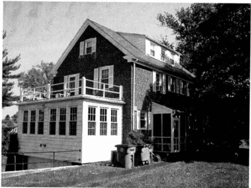
View from southwest showing enclosed porch above garage on west elevation
