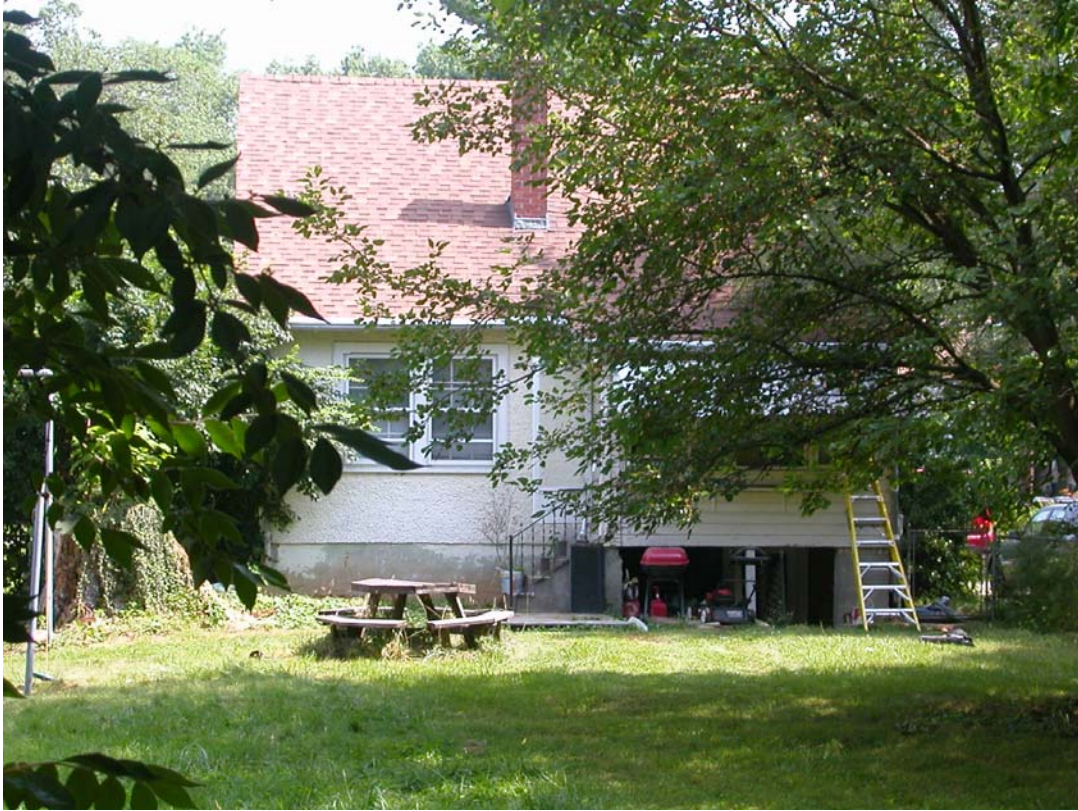
View of south elevation from alley
