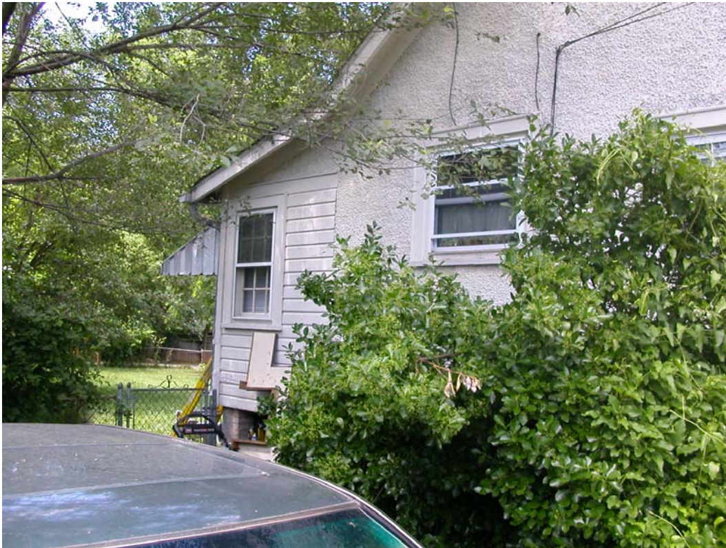
Detail of west elevation showing rear bump out
