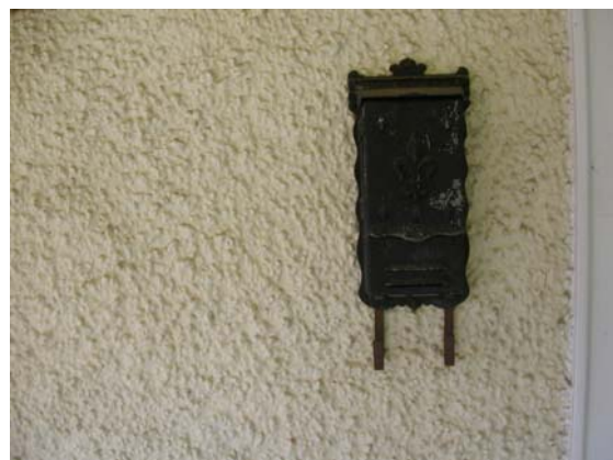
Detail of façade showing pebble-dash finish
