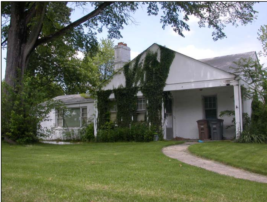
721 W. Montgomery Avenue, south elevation
