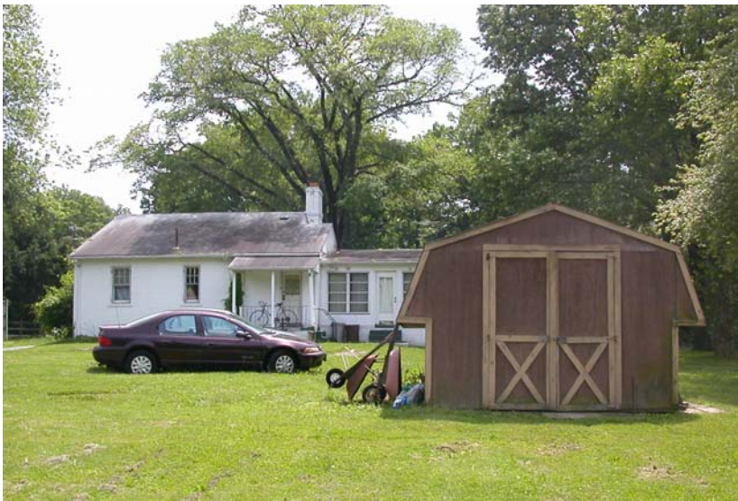
Shed, north elevation
