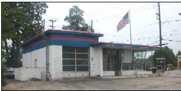
801 Hungerford Drive, west repair bay
