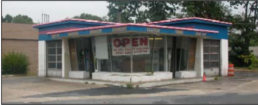
801 Hungerford, west (facing Hungerford Drive) and south elevations.
