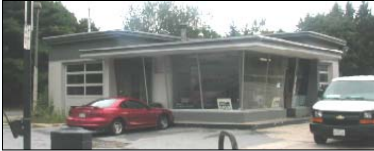
21615 Laytonsville Road, Laytonsville
