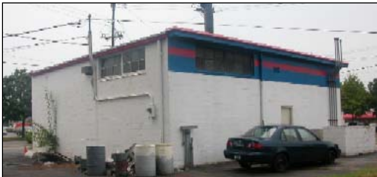
801 Hungerford, Rear (north and east) elevations.
