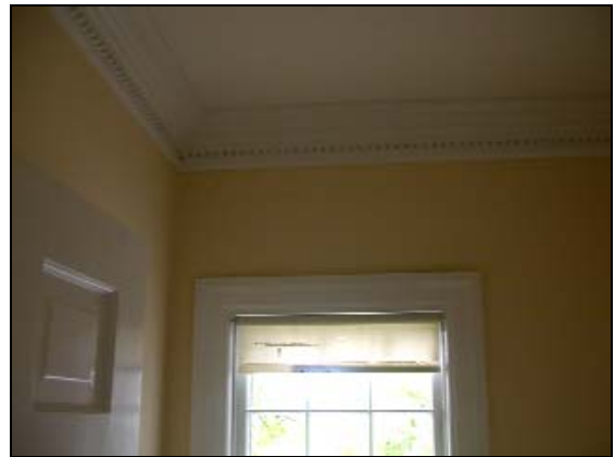
Guest bathroom, molding and window trim
