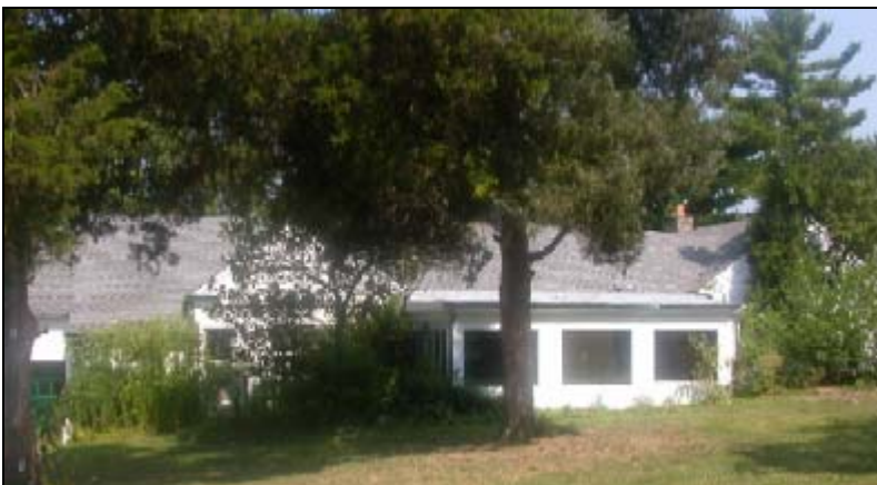
Rear elevation with sunroom addition.
