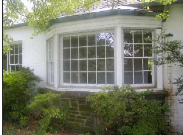
Façade bay window
