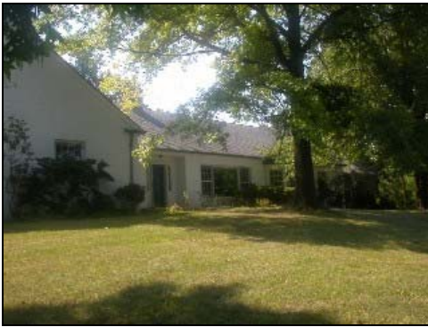
West façade, northern section
