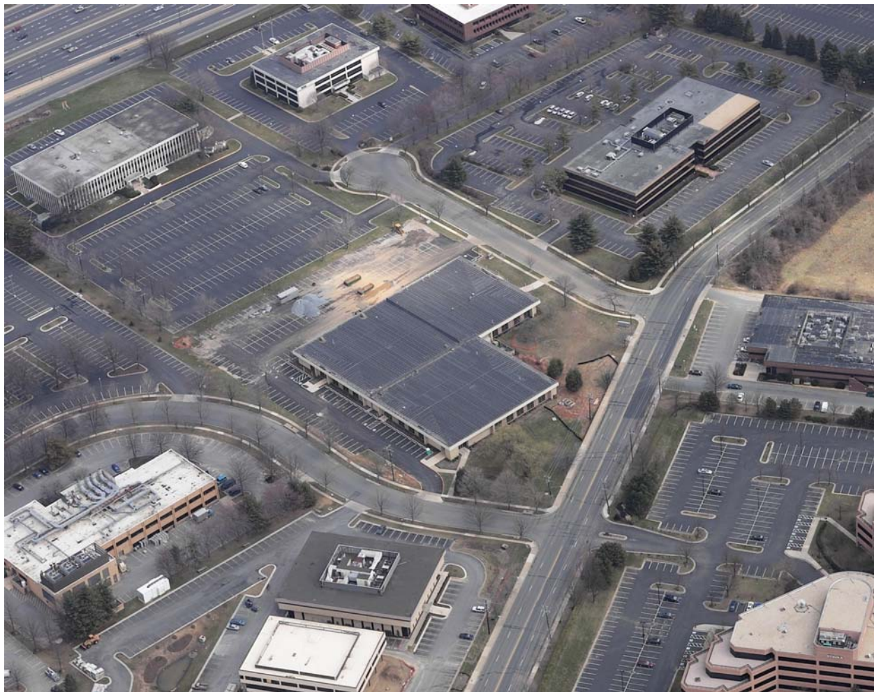
Aerial Overview of 4 & 5 Research Place
