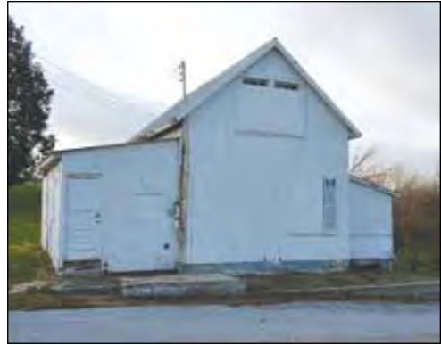
16100 Frederick Rd. ▲ 1930s King Farm Tenant House #8
