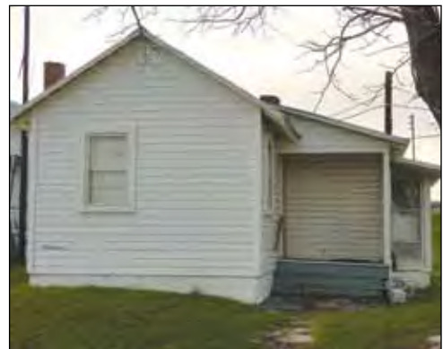
16100 Frederick Rd. ▲ 1950s King Farm Tenant House #7
