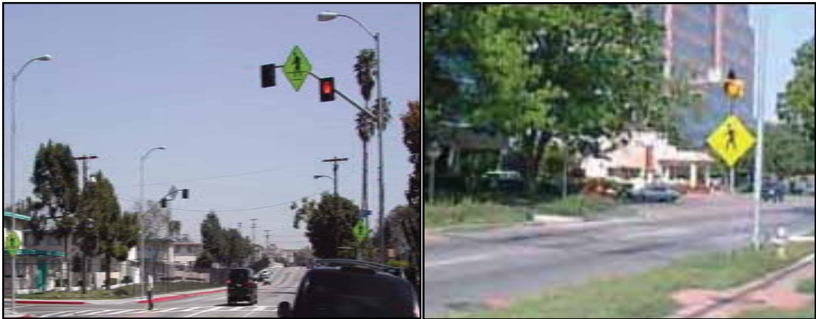
Figure 11 – Pedestrian Crossing Flashing Beacon
