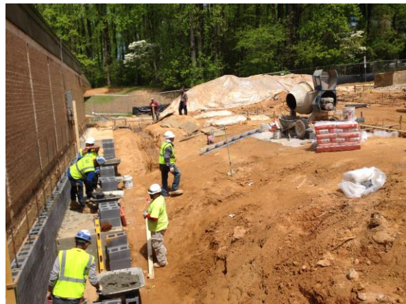
Block Installation
