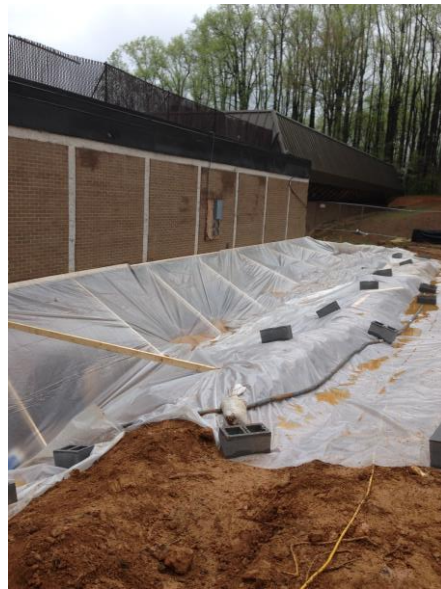
Protecting Exposed Areas During Rain
