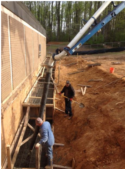
Concrete Placement
