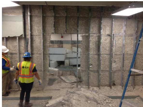
Locker Room Demolition
