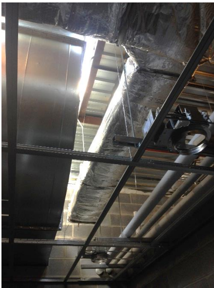
Duct and Ceiling Grid Installation
