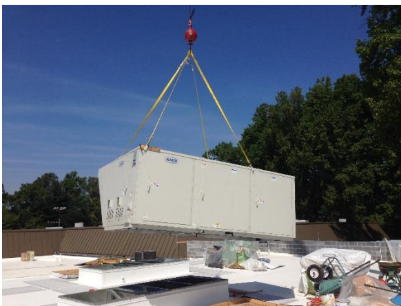
HVAC Roof-Top Unit Delivery
