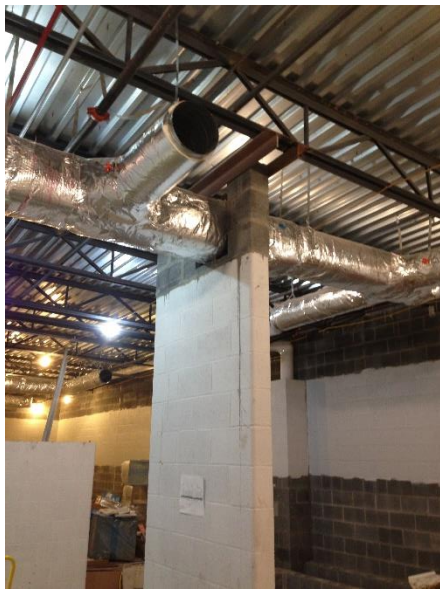
Duct and Partition Wall Installation
