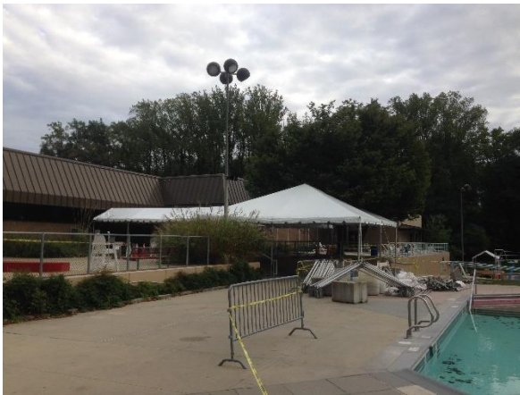
Covered Walkway Installation
