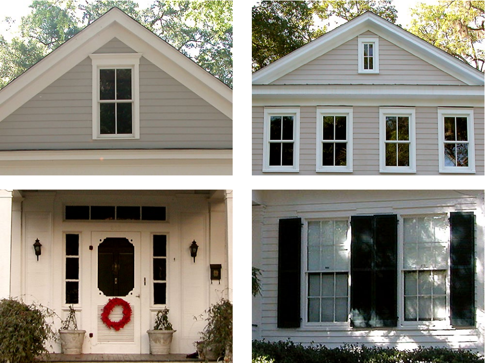
Typical Classical Vernacular doors & windows.
