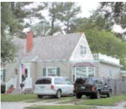
The side wing addition
