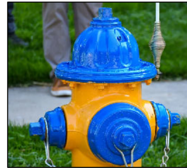
Sanitary sewer main with root in joint defect that requires rehabilitation (top); fire hydrant (bottom)
