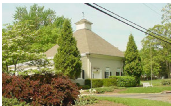
Figure 20. Croydon Park pumphouse
