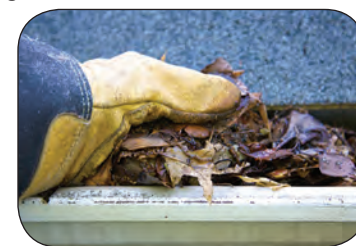
Gutters should be cleared out regularly to ensure proper conveyance of water.
