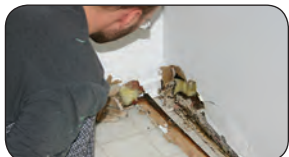
Repairing mold and water damage
