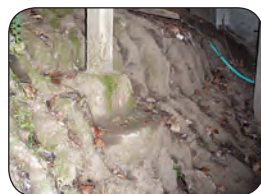
Visible erosion under a deck is common.
