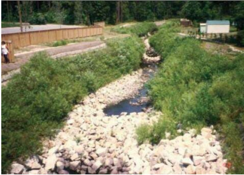
Priority 4 - Harden Channel in Place
