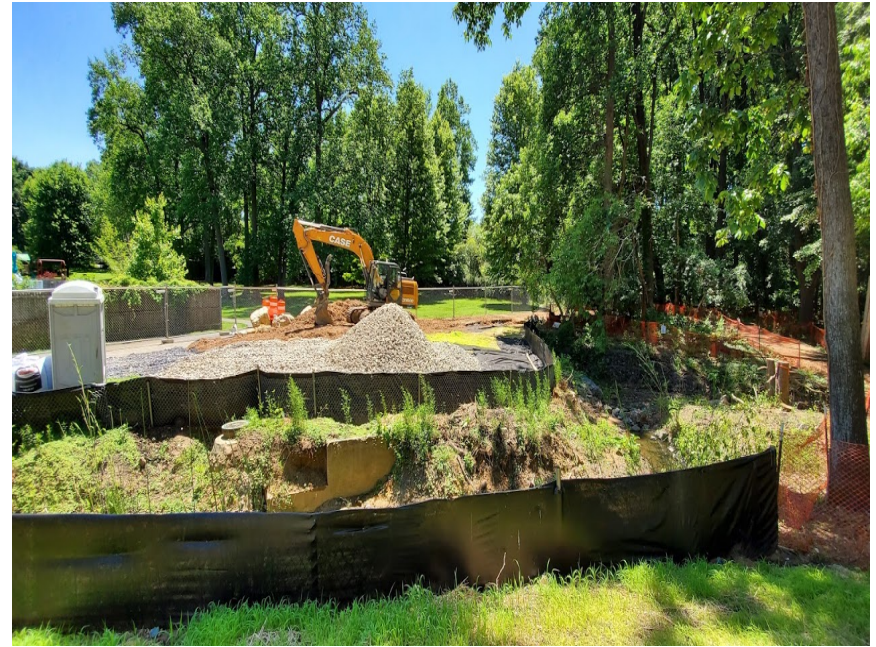
Staging and Stockpiling
