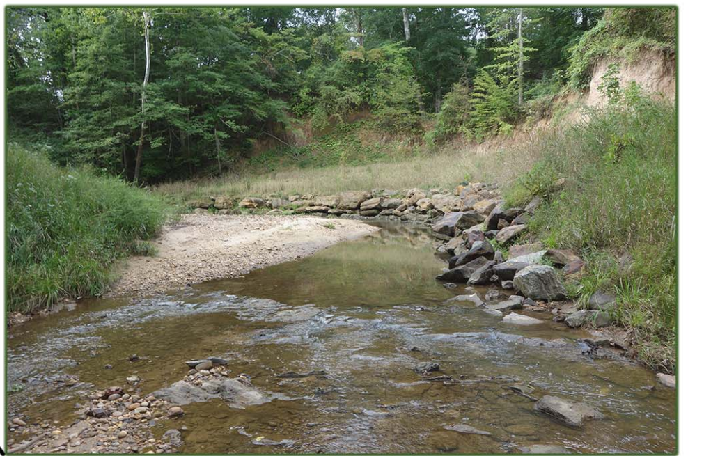
BOULDER REVETMENT EXAMPLE
