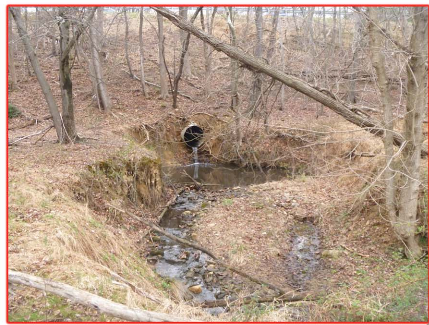
EXISTING OUTFALL & EROSION
