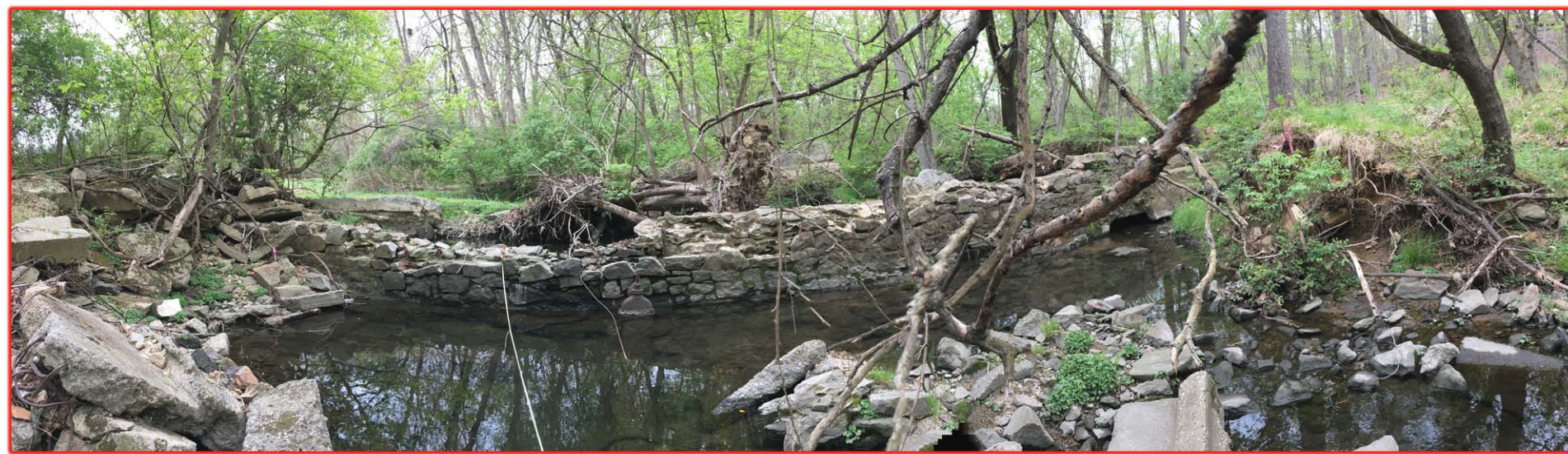
EXISTING DAM & INSTREAM RUBBLE TO BE REMOVED
