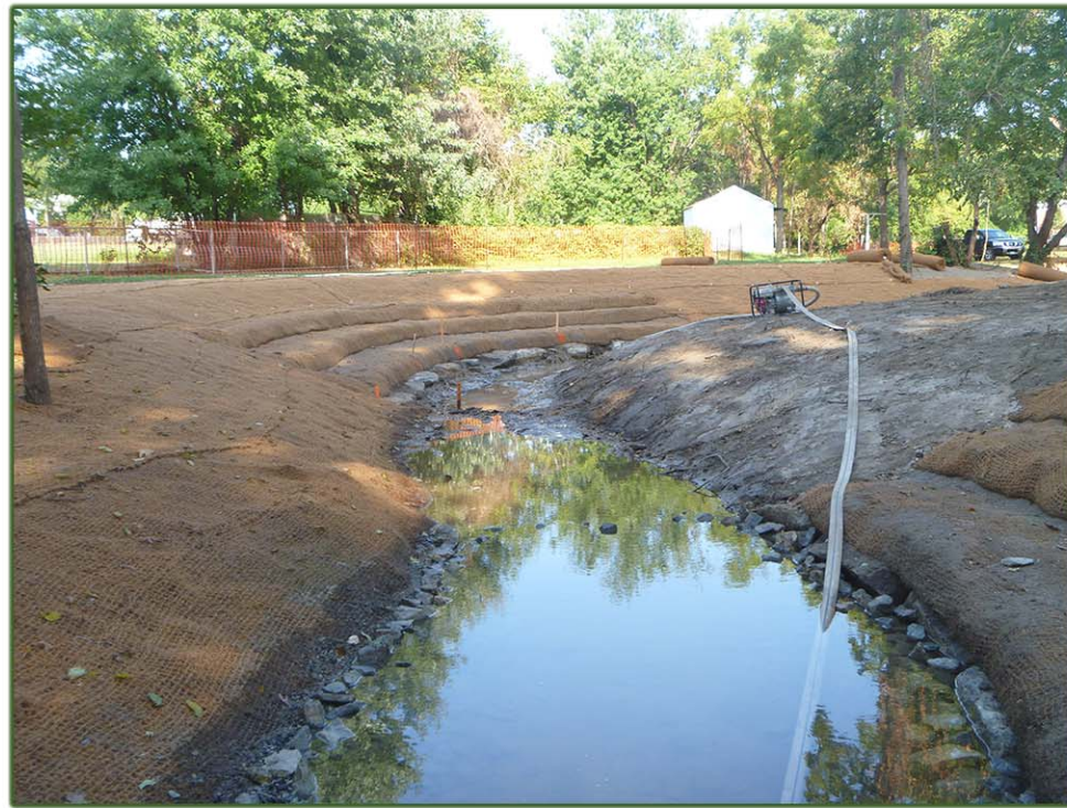
WRAPPED SOIL LIFT CONSTRUCTION EXAMPLE & PUMP DIVERSION
