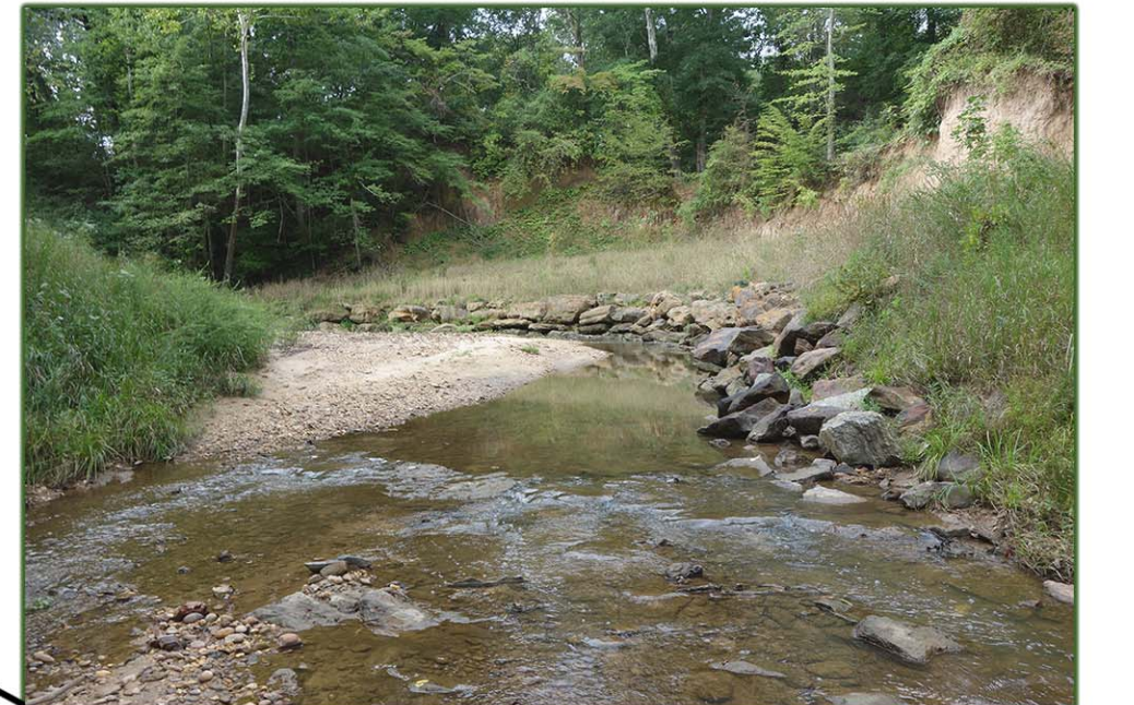
BOULDER REVETMENT EXAMPLE
