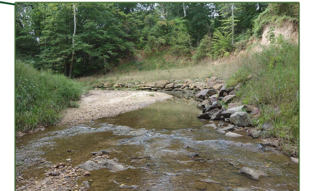
BOULDER REVETMENT EXAMPLE
