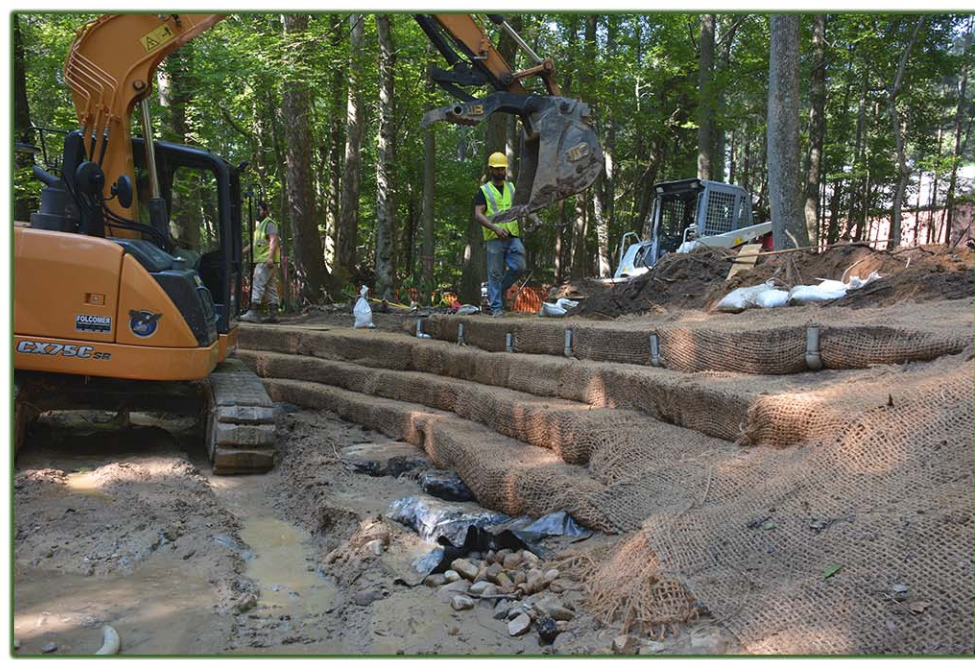
WRAPPED SOIL LIFTS CONSTRUCTION EXAMPLE
