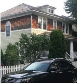
Horizontal band, materials change between stories.
