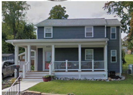
Set back addition, matches colors & detail, roof ridge & eave lower than those of the original structure.
