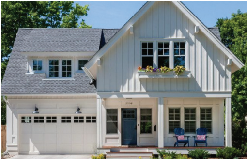
Garage beside house, set back.
