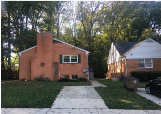
Side entry turned away from the street.
