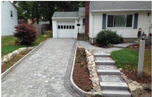
Driveway with pervious materials.
