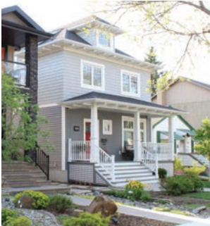
Horizontal band, materials change between stories.
