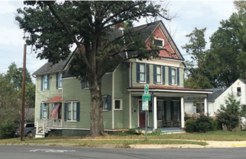
Corner House, articulated both façades.
