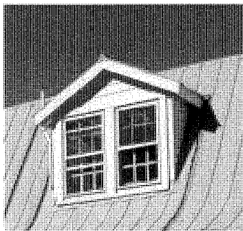
South Gabled Dormer
