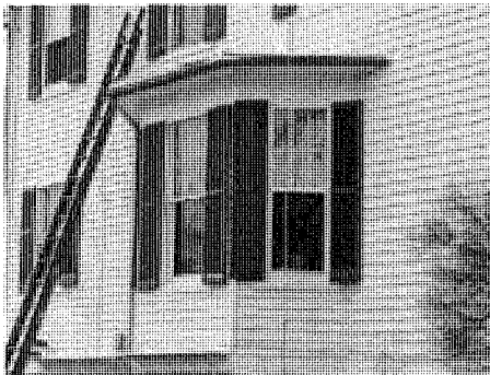
BAY WINDOW, EAST FACADE
