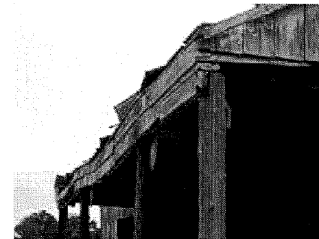
Condition of plates
