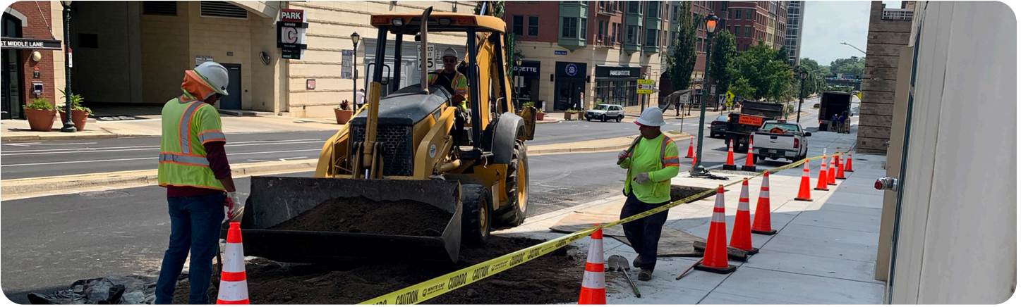
Construction workers widen the sidewalk along E. Middle Lane in Rockville Town Center.
