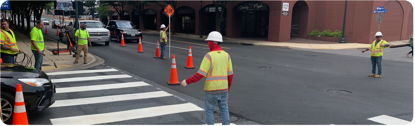
A construction crew installs a marked crosswalk and helps direct motorists along North Washington Street.
