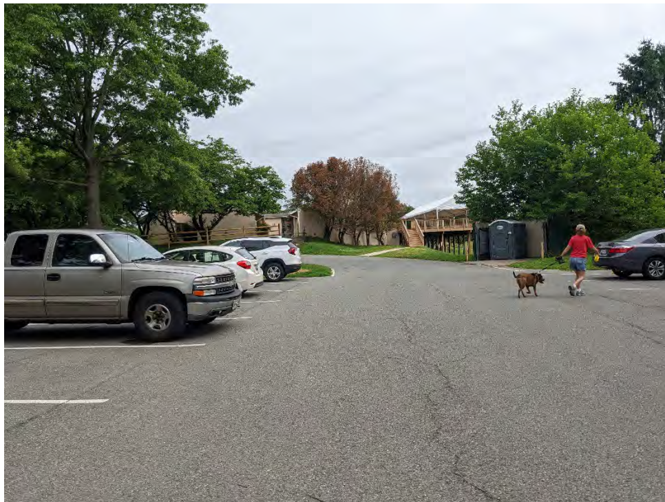
Figure 51: Minor Pavement Cracks within Parking Lot
