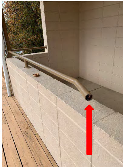
Fig. 16: Existing Tube Railing
