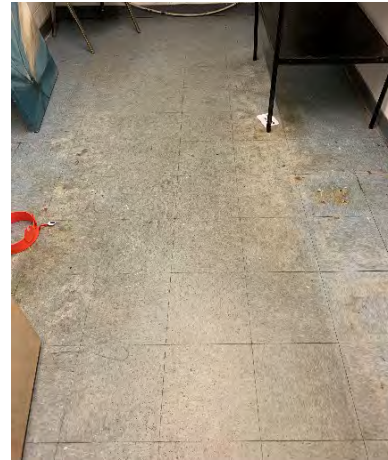
Fig 19: Typical Floor Tile
