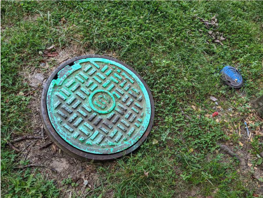
Figure 34 : Water Valve and Sanitary Sewer Manhole West of the Building
