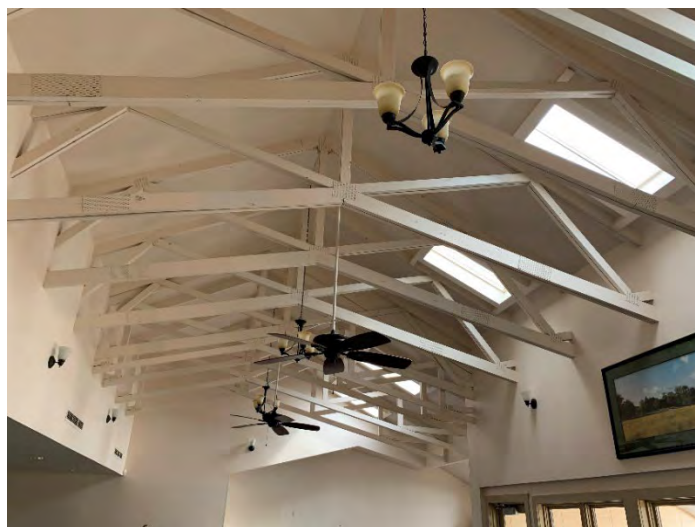
Fig. 25: Exposed Truss Ceiling with Gypsum Board
