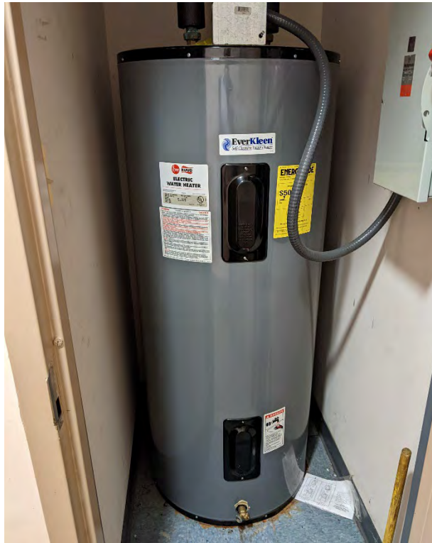
Figure 46: Electric Storage Water Heater
