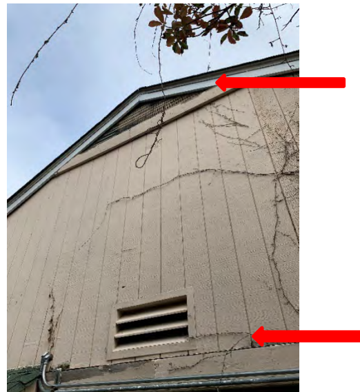
Figure 6: South Wall T-111
