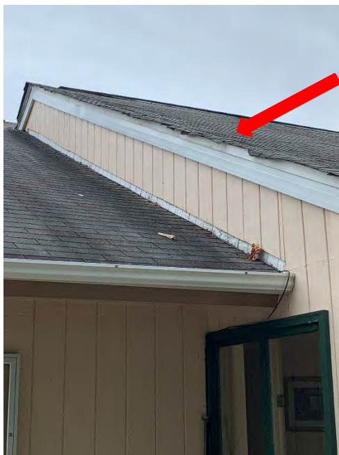
Fig. 12: Roof End Conditions on West Roof
