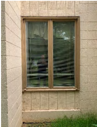
Figure 9: Original Single-Pane Casement Window
