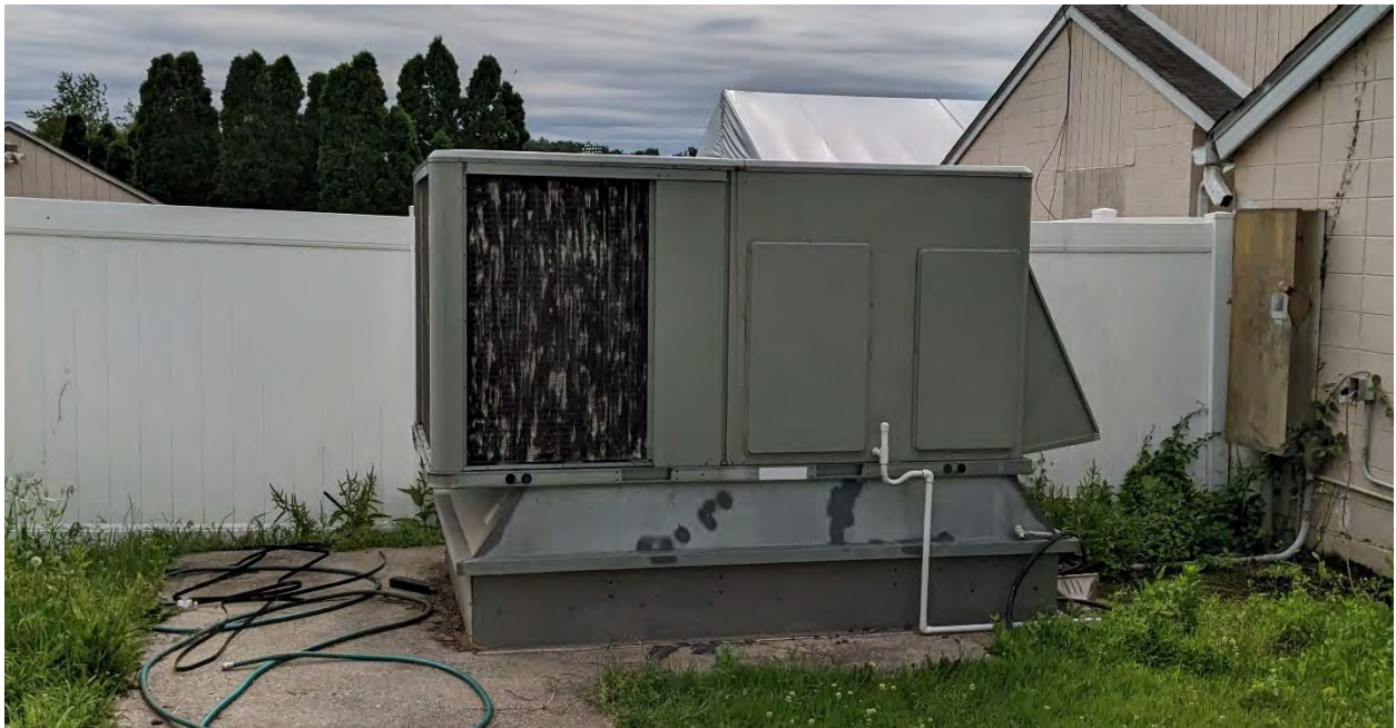
Figure 42: Packaged RTU
