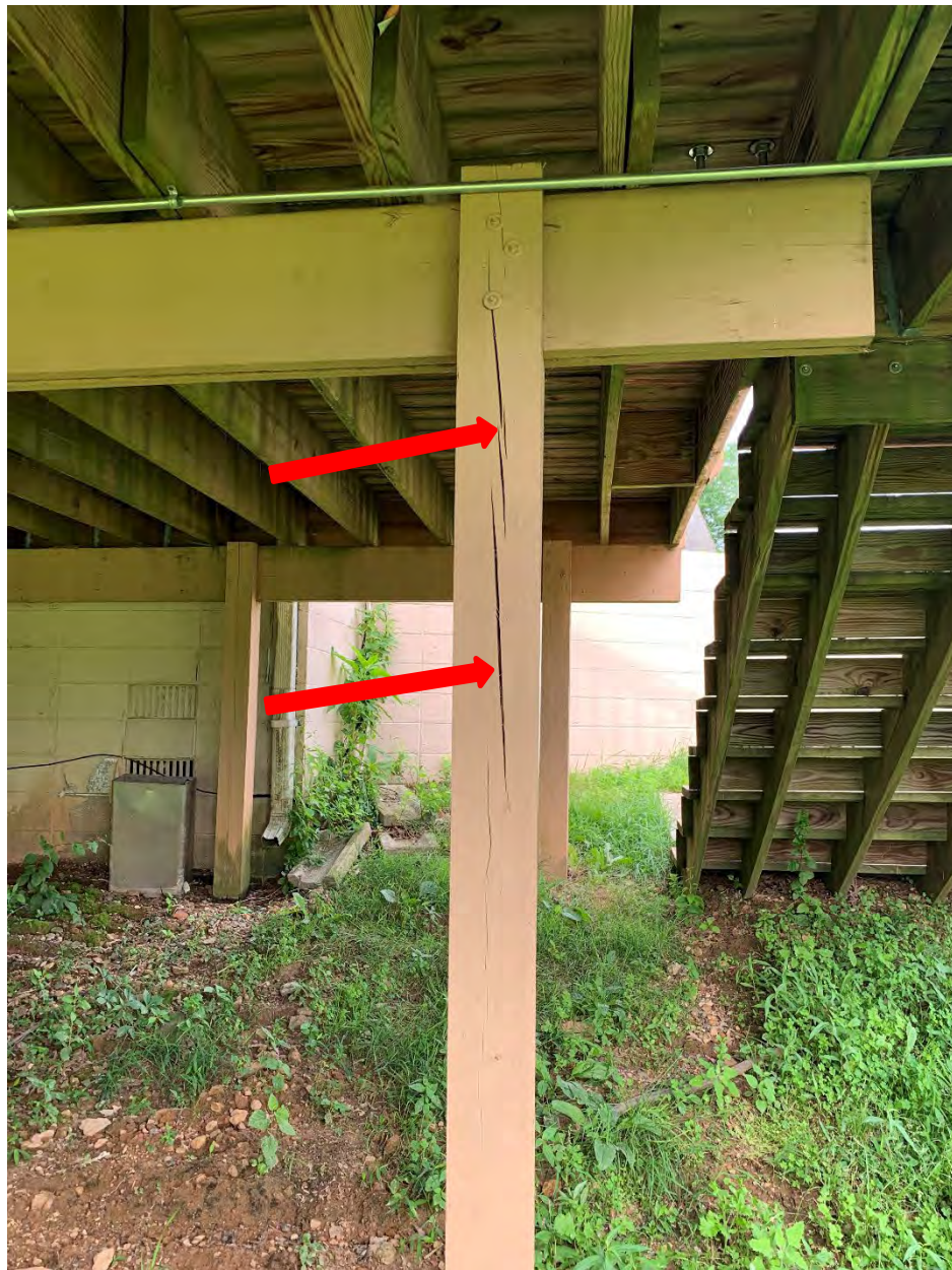
Figure 38: Vertical Checks at Deck Posts
