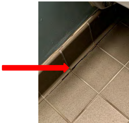
Fig. 29: Separation of Floor
