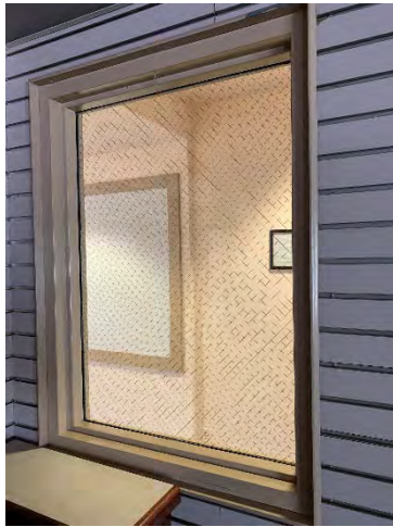
Fig. 26: Wire Glass Interior Window
