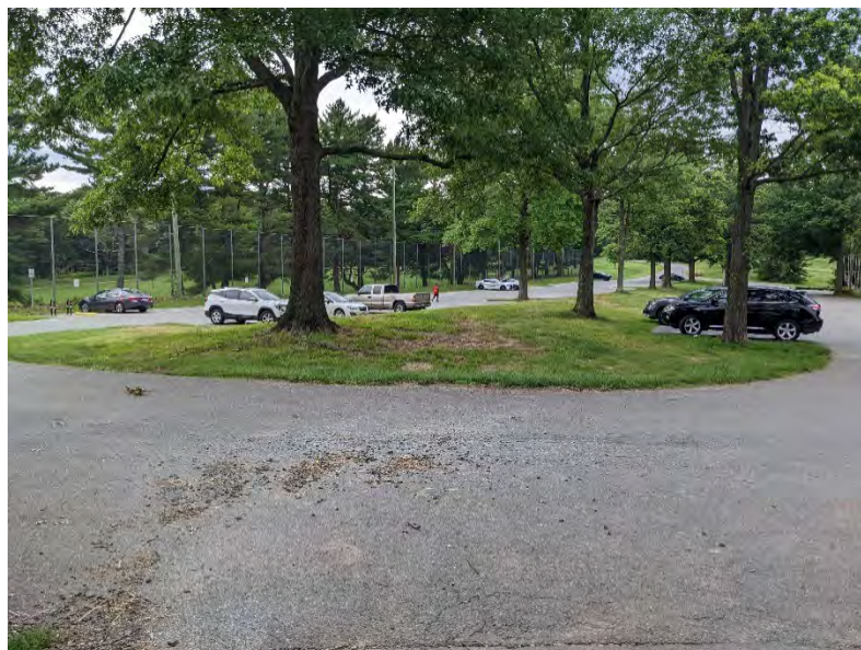
Figure 50: Parking Lot from top of Drop-off Loop
