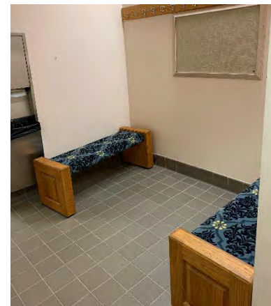
Fig. 21: Typical Toilet Room Tile
