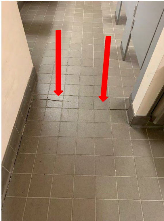
Figure 35: Change in Floor Elevation at Women's Bathroom
