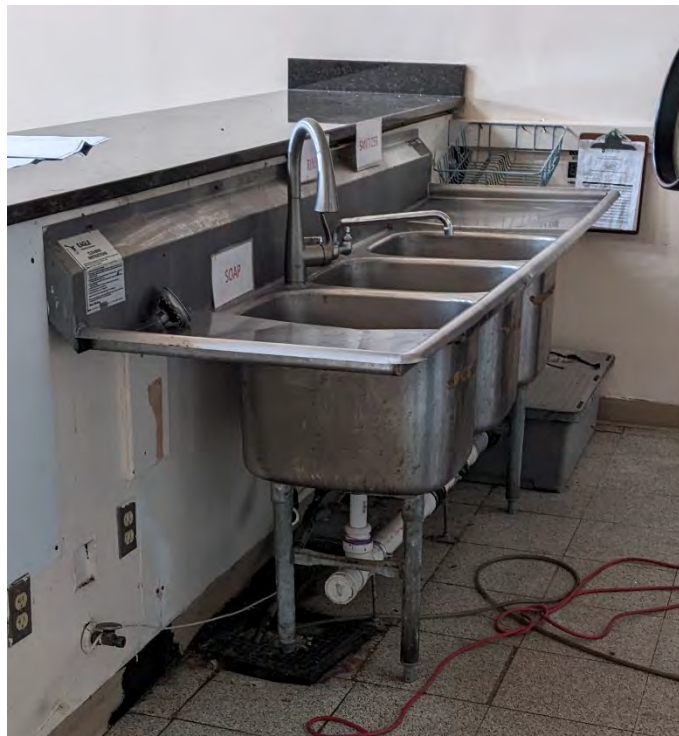
Figure 48: Three-Compartment Sink with Floor-mounted Grease Interceptor
