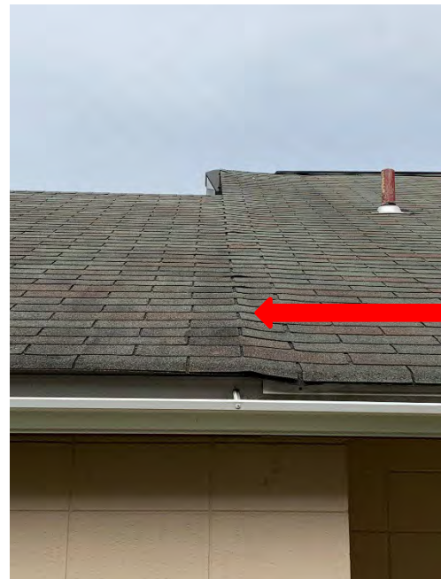
Fig. 13: Warping of Roof Plane
