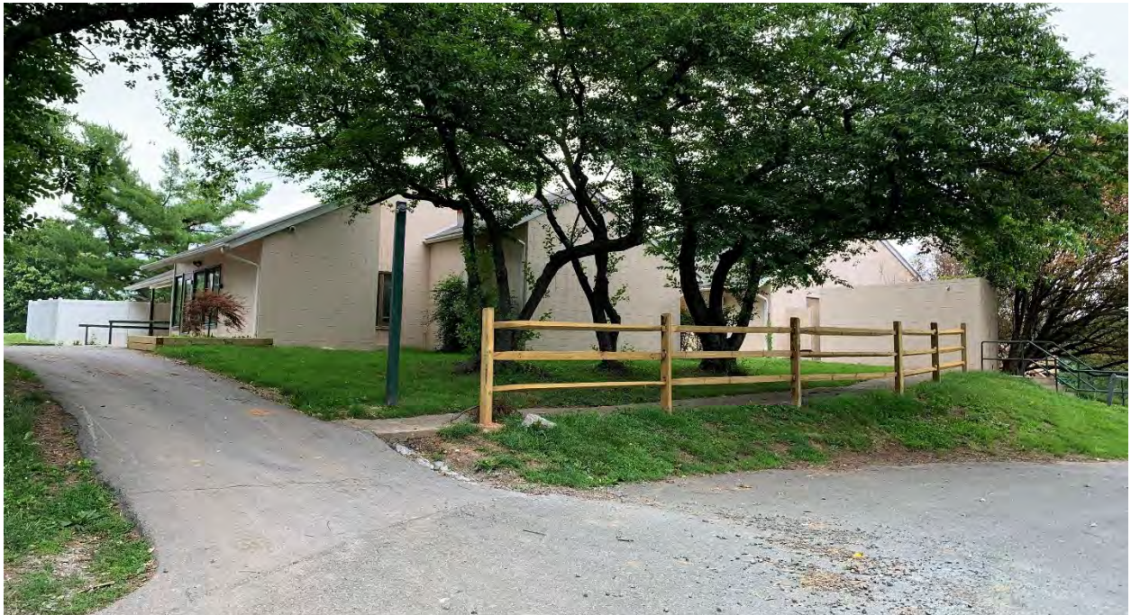
Figure 1: Clubhouse, South Elevation, June 2022
