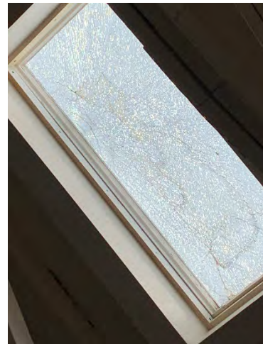
Fig. 28: Broken Skylight
