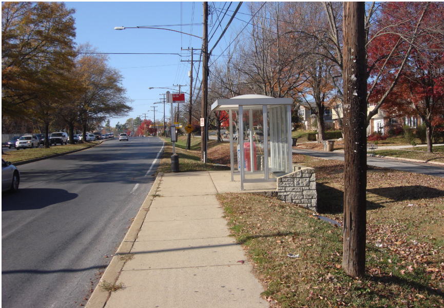
Bus shelter on Veirs Mill Road
