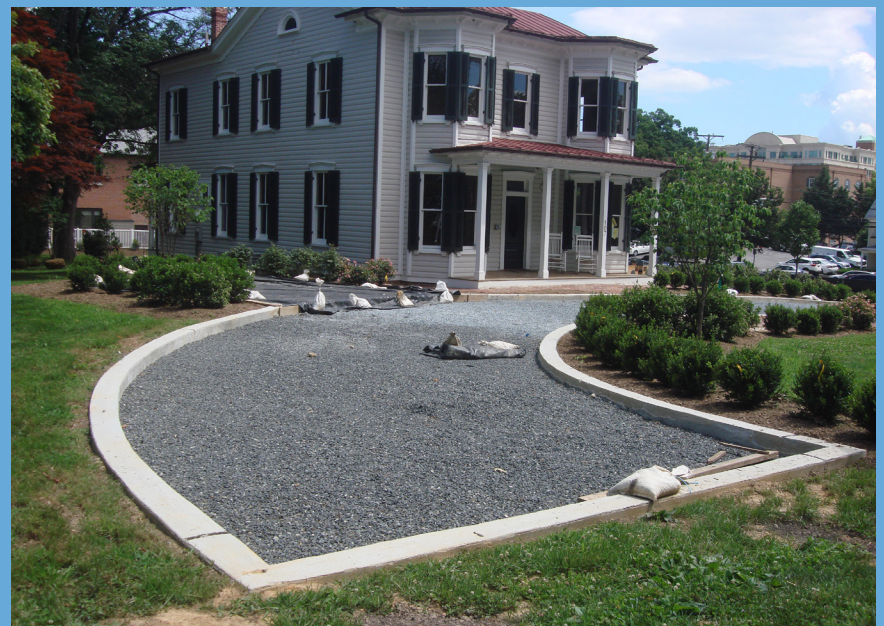
An historic house on West Jefferson Street installed a permeable paver driveway in 2018, shown here during construction of the gravel subsurface.
