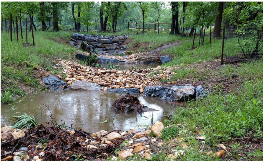
Step pools were installed in Dogwood Park to retain and slow water in a series of steps as water flows from an outfall into a tributary of Cabin John Creek. The project also restored highly eroded stream banks. Slowing and retaining water behind the steps reduces the flash speed of runoff when it rains, which helps to protect banks from future erosion.
