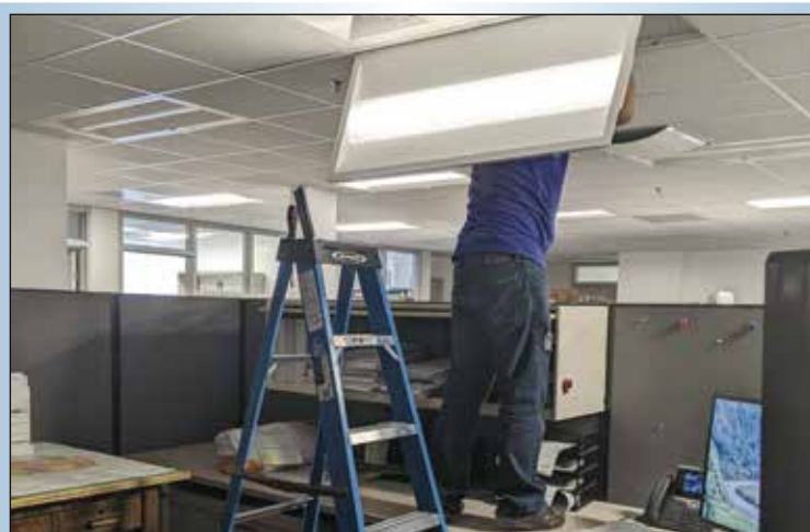
CITY HALL, IN A NEW LIGHT ... Contractors in March installed new energy-efficient light-emitting diode, also known as LED, lights with occupancy sensors at City Hall. The project upgrades 325 interior light fixtures on the second floor, including 256 sensors to reduce energy costs, maintenance and greenhouse gas emissions. Funding for the project leverages a $35,000 grant from the Maryland Energy Administration and Pepco utility rebates to work towards the Mayor and Council's goals of leading by example to reduce energy consumption and greenhouse gas emissions from municipal facilities.
