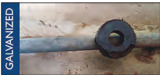
Grey or silver, and a magnet sticks to it: You have a galvanized steel service line.
