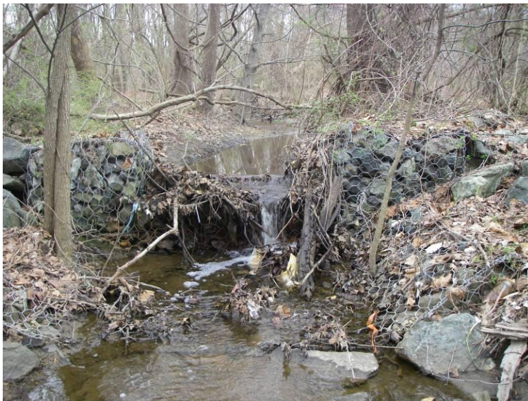
FIGURE 45: IN-STREAM GABION WEIR (REACH SLT-005)
