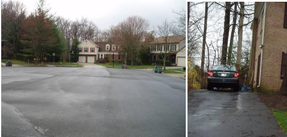
FIGURE 19: EXCESSIVELY WIDE CUL-DE-SAC (N-101); DOWNSPOUT INDIRECTLY CONNECTED TO THE STORM DRAIN (N-102)
