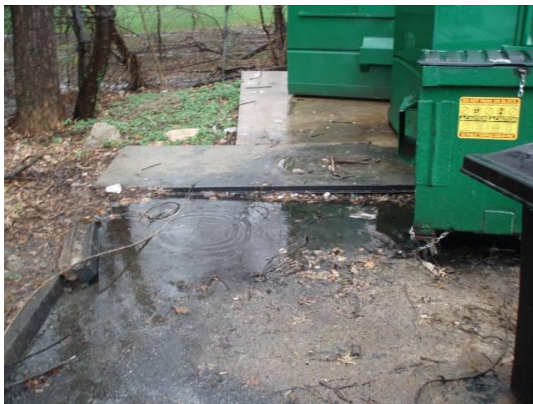
FIGURE 42: OVERFLOWING GREASE TRAP (H-302).
