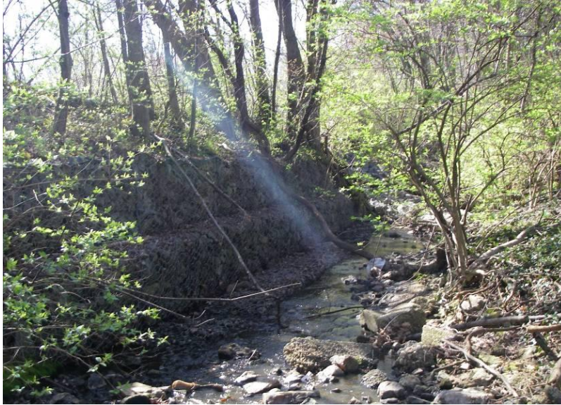
FIGURE 29: STREAMBANK ARMORING (REACH EST-001)
