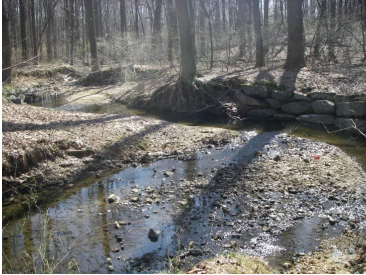
FIGURE 14: RIP-RAP ARMORING (REACH BOG-004)
