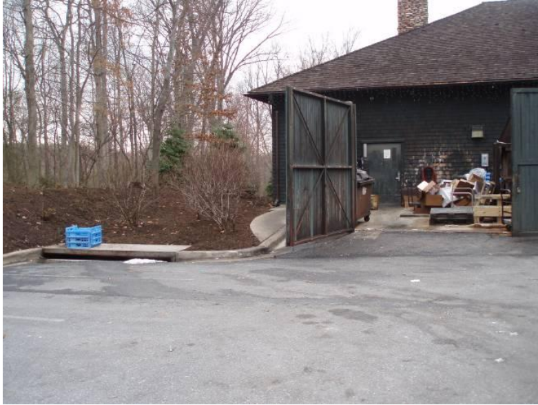
FIGURE 25: EVIDENCE OF WASHWATER DUMPING INTO STORMDRAIN SYSTEM (H-308)
