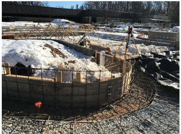
Activity Pool Walls Preparations
