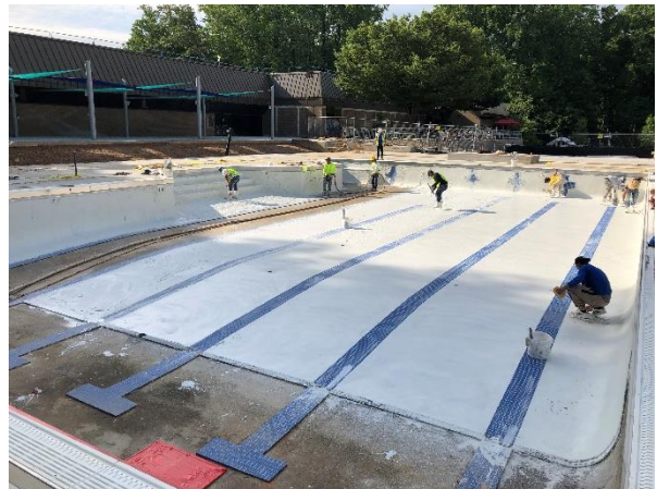
Pool Plaster Installation
