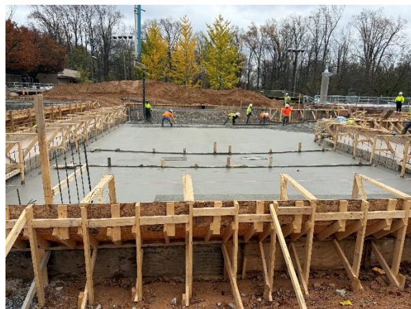
Activity Pool Concrete
