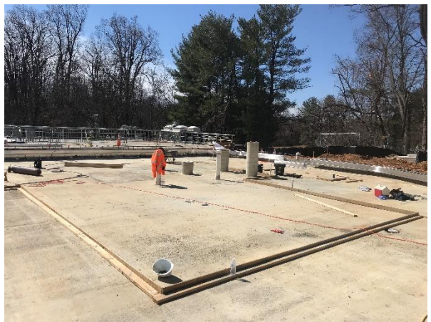
In-Water Play Unit Supports
