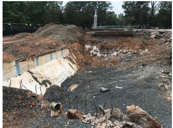
1968 Pool Shell Removal
