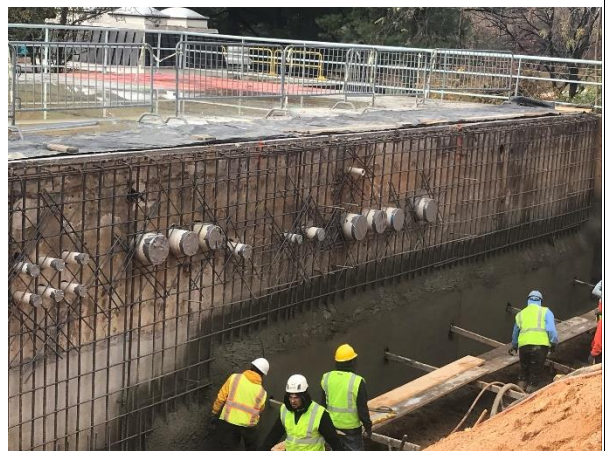
Filter Room Wall
