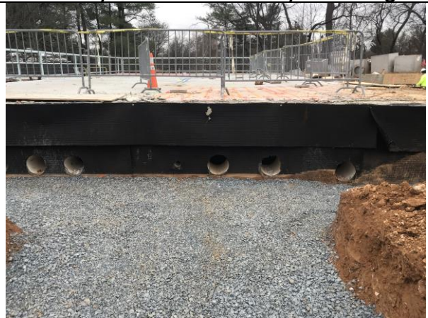
Pool Pipe Sleeves into Filter Room
