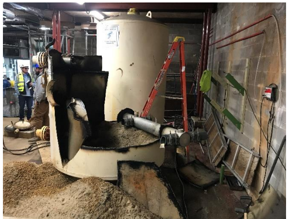
Removal of Old Pool Filter Equipment
