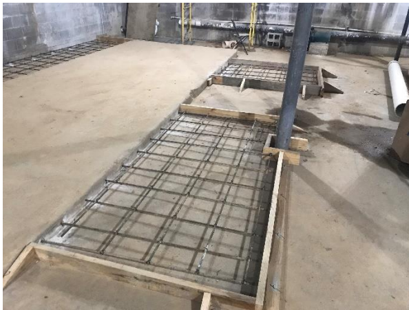
Pump Room Floor Preparations
