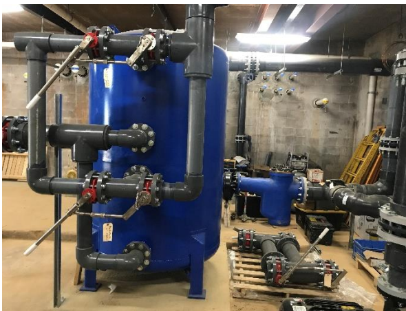
Filter Tank Installation
