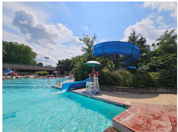
Water Slide (pre-construction)
