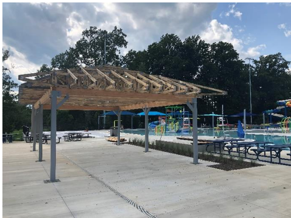
Picnic Pavilion Installation
