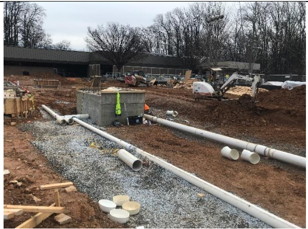
Pool Water Surge Chamber
