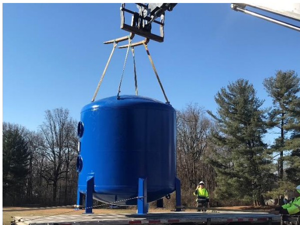
Filter Tank Delivery
