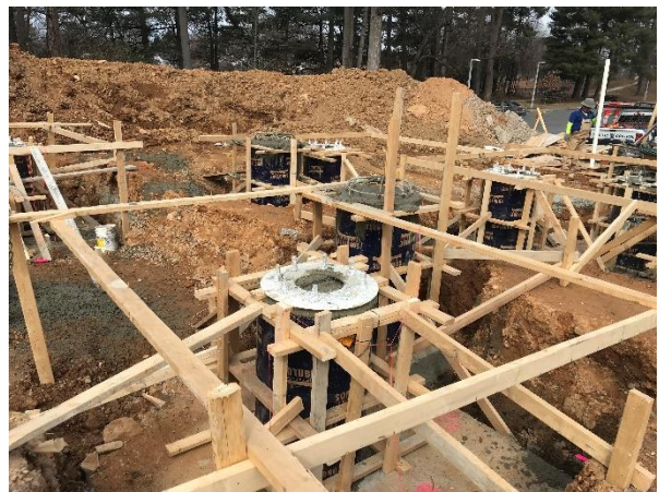
Water Slide Structure Footers
