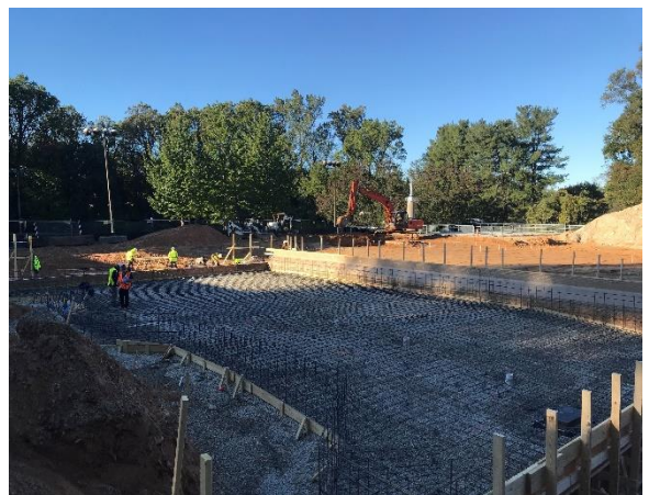
Wellness Pool Prior to Concrete
