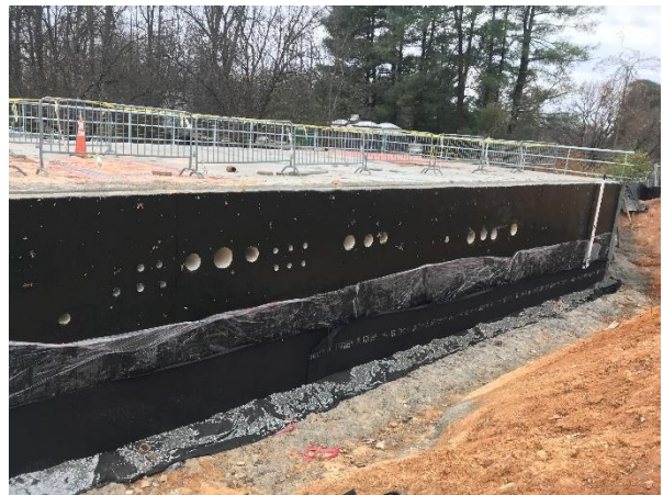
Filter Room Wall Waterproofing
