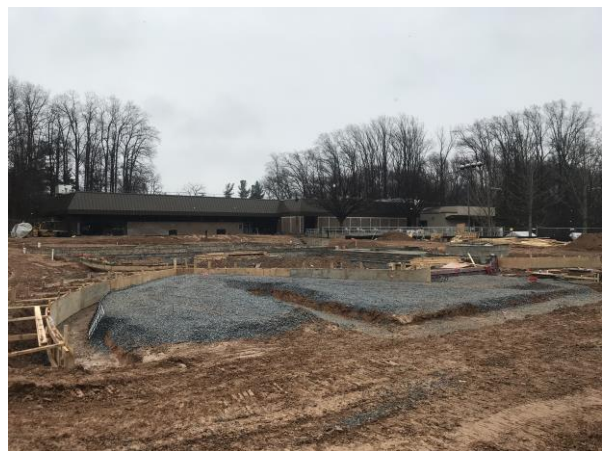
Activity Pool "Beach Entry" Grading
