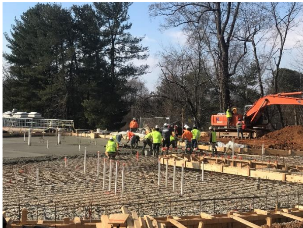
Activity Pool Floor Concrete
