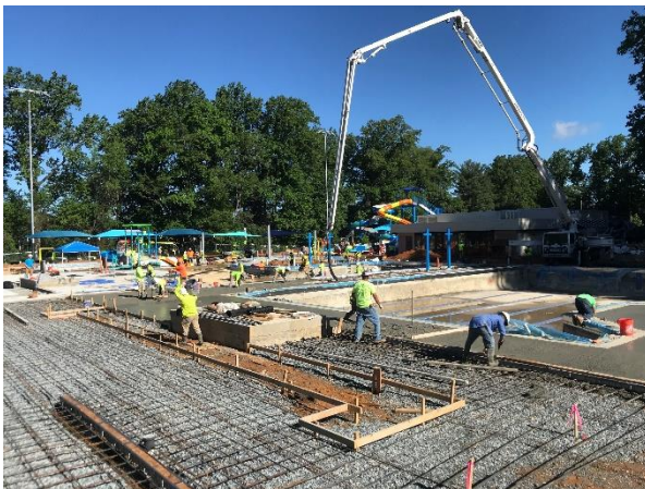
Concrete Pool Deck Installation
