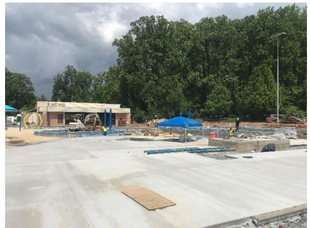
Concrete Pool Deck
