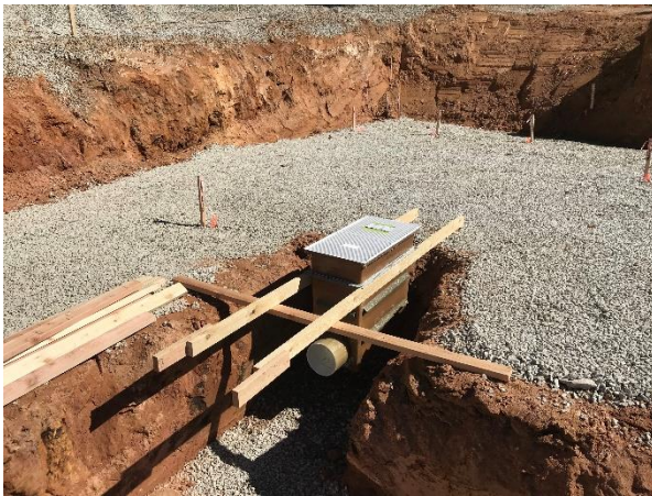
Setting Wellness Pool's Main Drains
