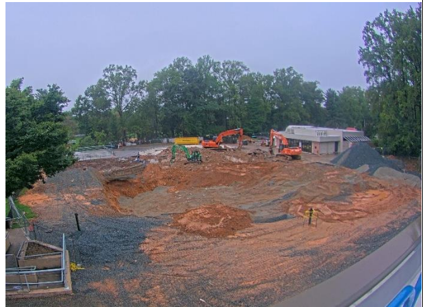
Sept. 27 Site Overview
