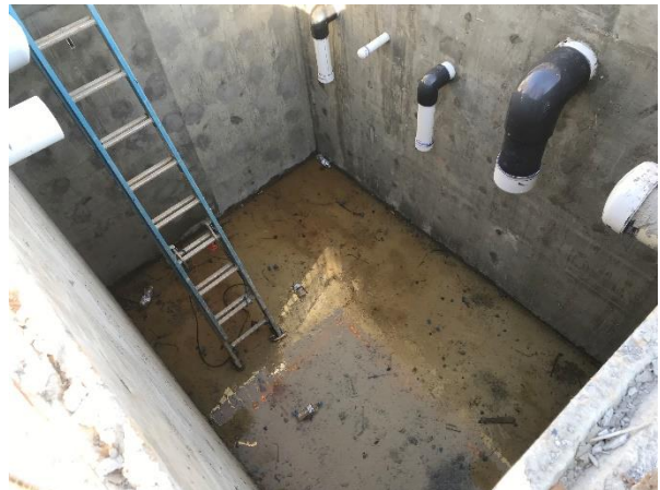
Water Slide Balance Tank
