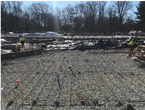
Activity Pool Floor Preparations
