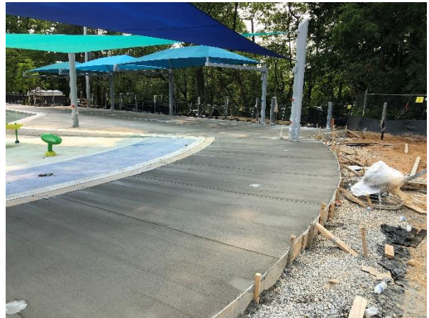
Pool Deck Concrete
