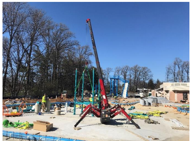
In-Water Play Unit Installation
