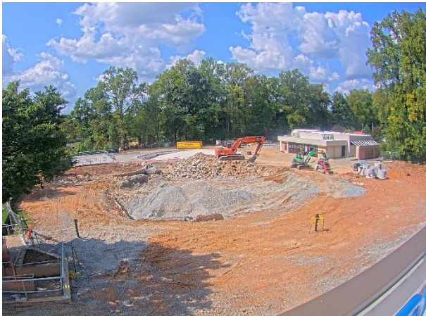
Sept. 20 Site Overview
