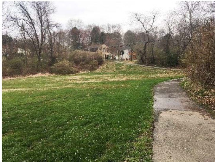
Drainage over pathway; saturated turf
