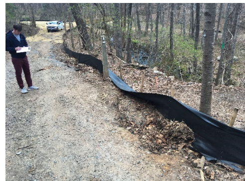
Severely Eroded Section under Restoration
