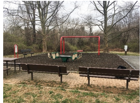
Drainage Issues at Playground Seating Area
