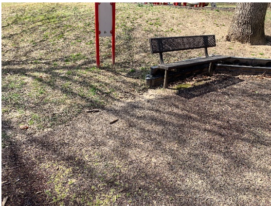
Soil Washed in Playground Surface
