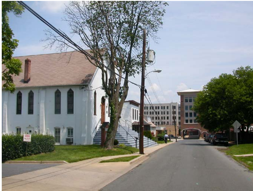
19 th century African-American church and parsonage adjacent to 21 st century Town Center
