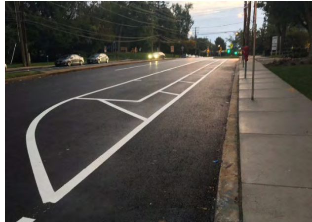
Figure 17. Example image of a buffered bike lane with parking. (Credit: The WashCycle)
