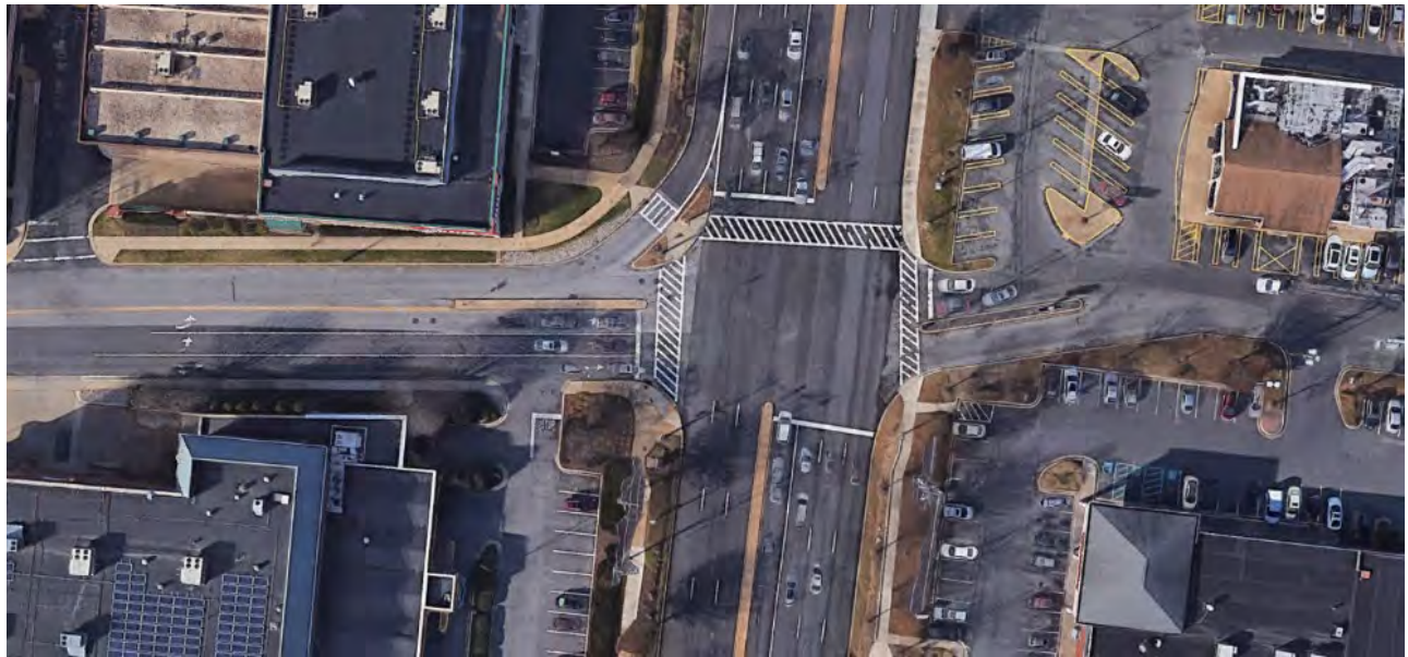
Figure 45. Existing Condition at MD 355.
