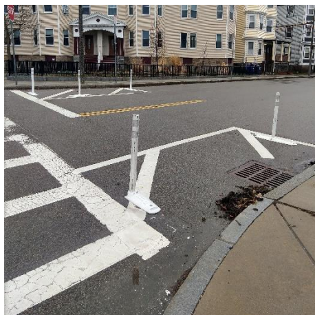
Daylighting; Double Yellow Centerline Striping
