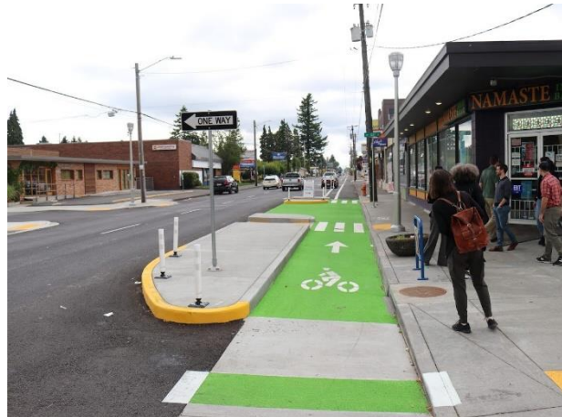
Curb Extensions with Bicycle Treatments
