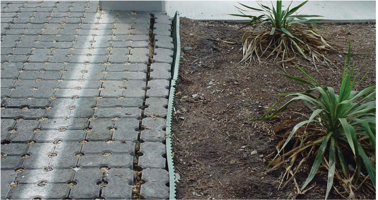
Failing edge restraint caused by improper product and installation
