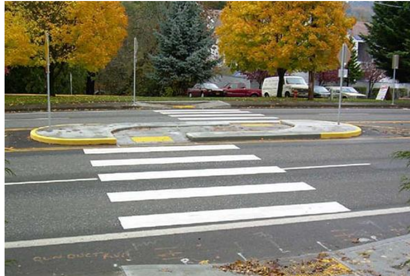
Permanent Pedestrian Refuge
