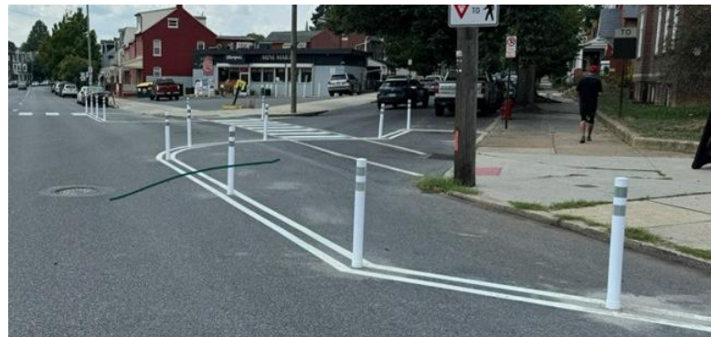
Painted Curb Extension and Flex Posts
