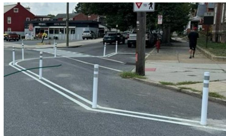
Painted Curb Extension and Flex Posts
