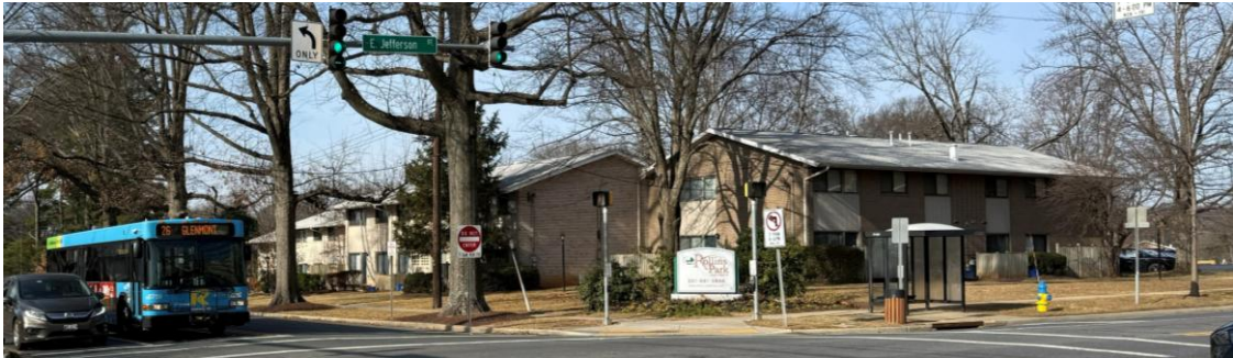
Transit on E Jefferson Street
