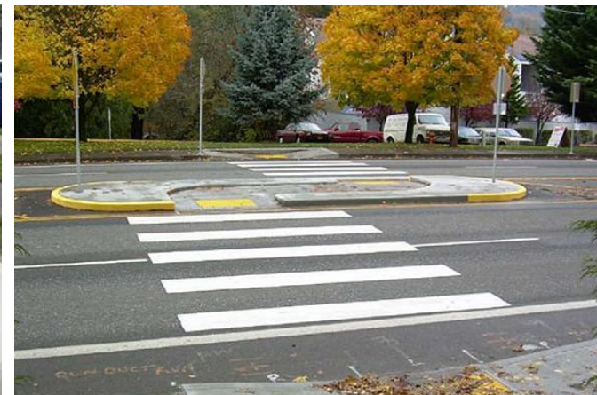
Concrete Pedestrian Refuge
