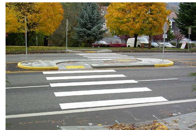
Concrete Pedestrian Refuge
