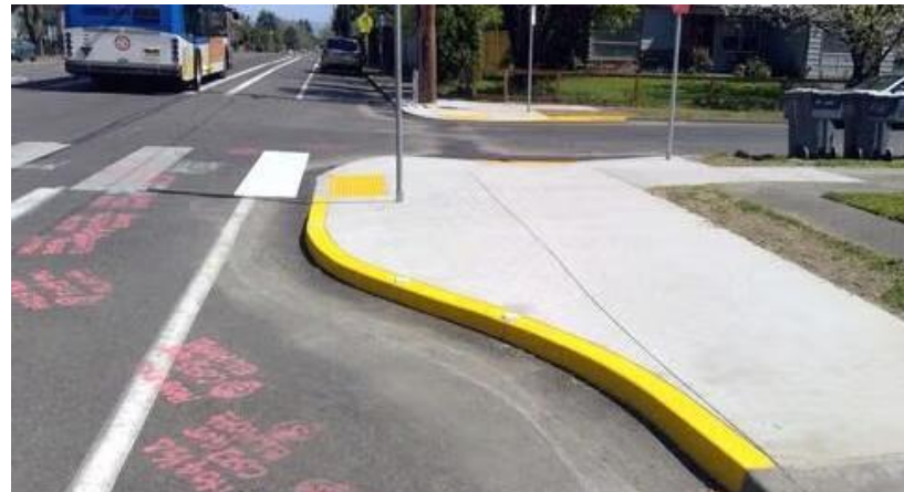
Concrete Curb Extensions
