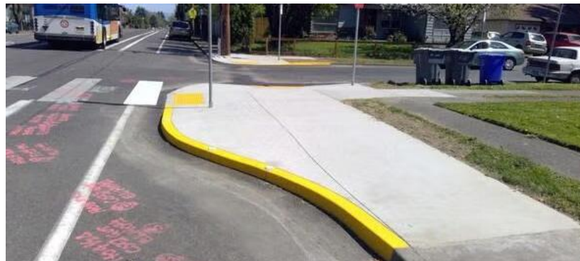
Concrete Curb Extensions
