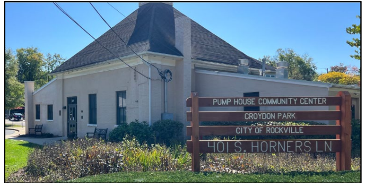
Pump House Community Center 401 S. Horners Lane | Rockville, MD 20850
