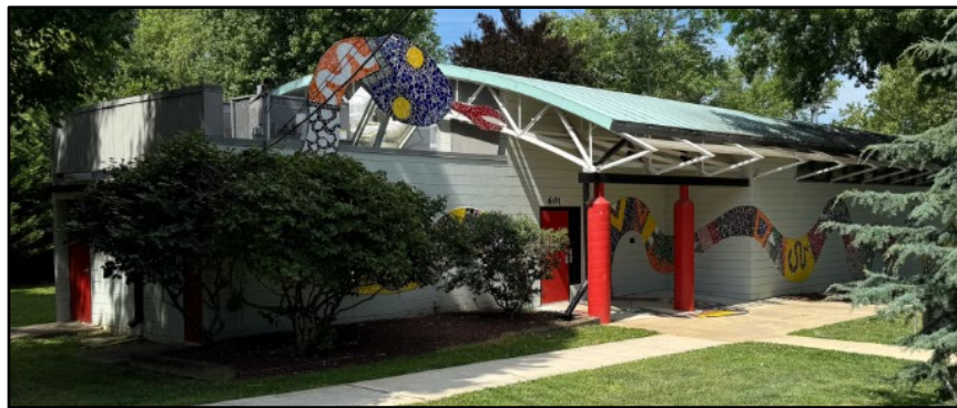
Elwood Smith Community Center 601 Harrington Road | Rockville, MD 20850
