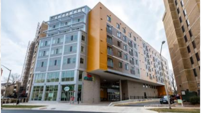
Main Street Apartments 70 units ( Built 2020 )
