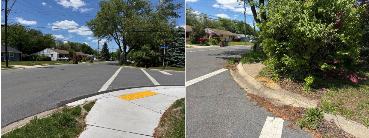
Figure 19. Lewis Avenue and Brooke Drive intersection with overgrown vegetation (looking north)
