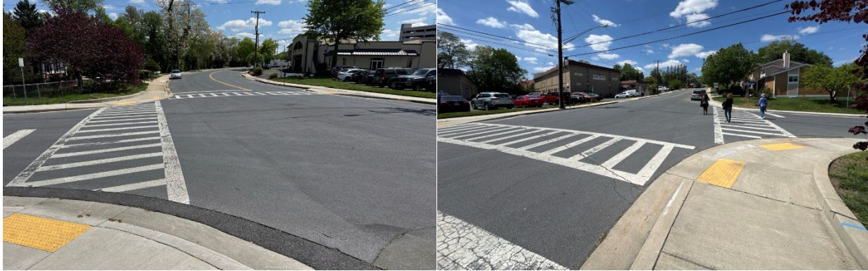
Figure 16. Lewis Avenue and Rockland Avenue intersection (left, looking south; right, looking north)
