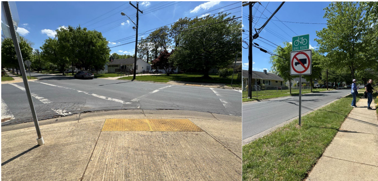
Figure 35. Lewis Avenue and Broadwood Drive intersection (left: looking south; right: looking north)
