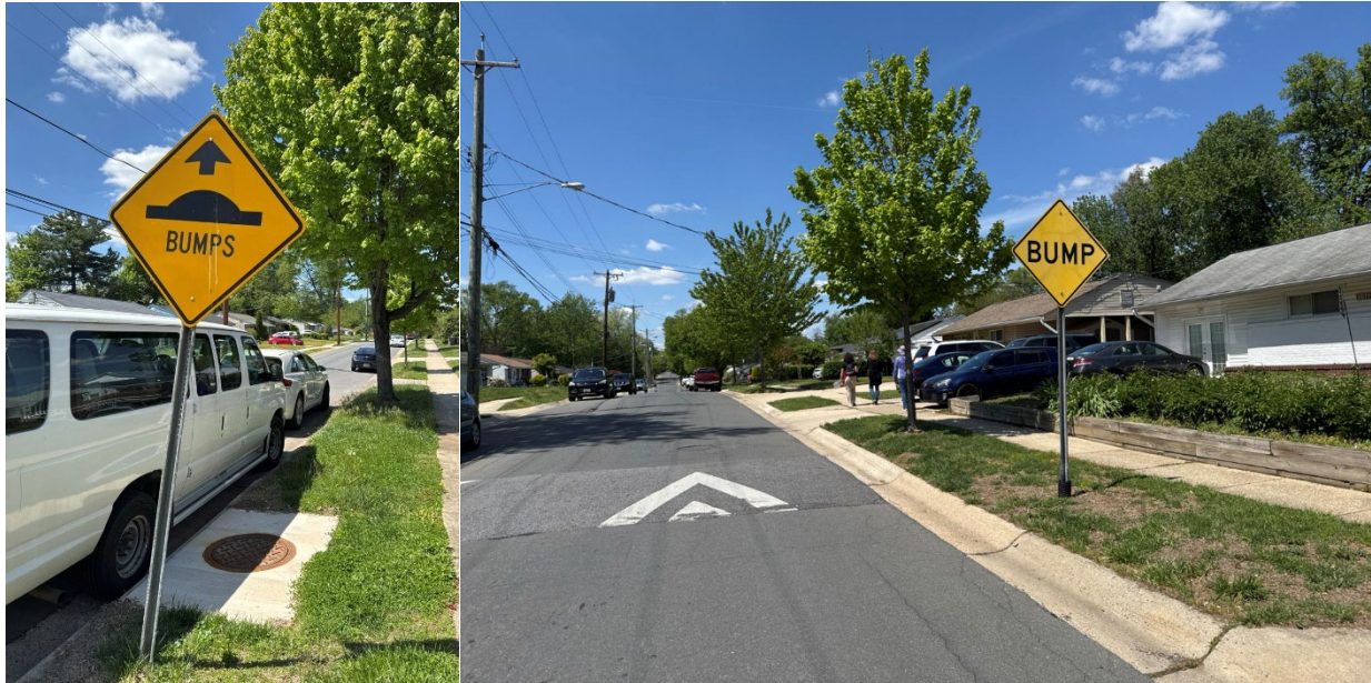
Figure 24. Signs and speed hump on Lewis Avenue between Matthews Drive and Thornden Road (looking north)
