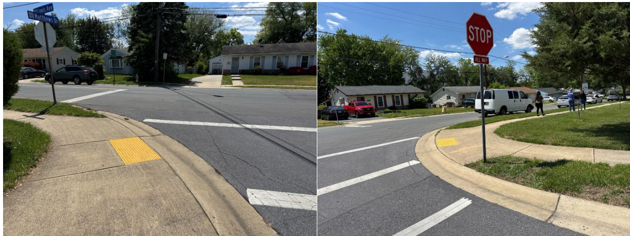
Figure 22. Lewis Avenue and Matthews Drive intersection (left, looking south; right, looking north)
