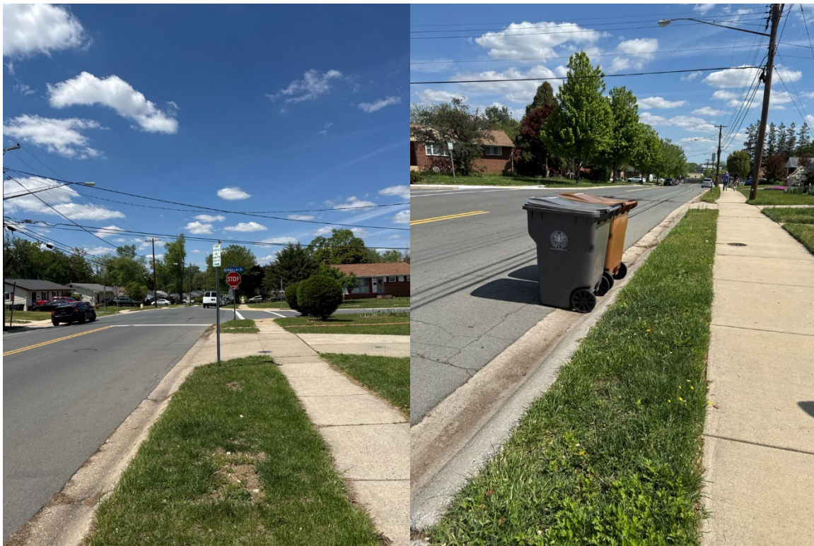
Figure 21. Lewis Avenue between Brooke Drive and Matthews Drive (left, looking north; right, looking south)
