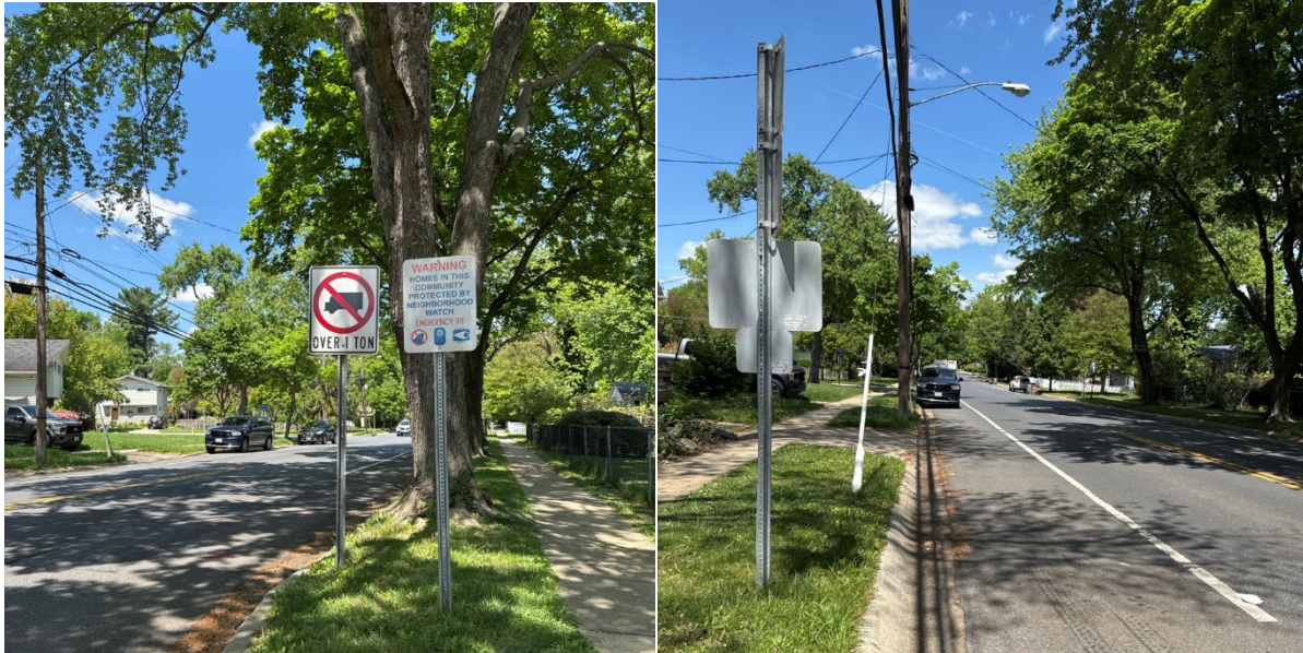
Figure 52: Ardennes Avenue between Halpine Road and Holland Road (looking north)
