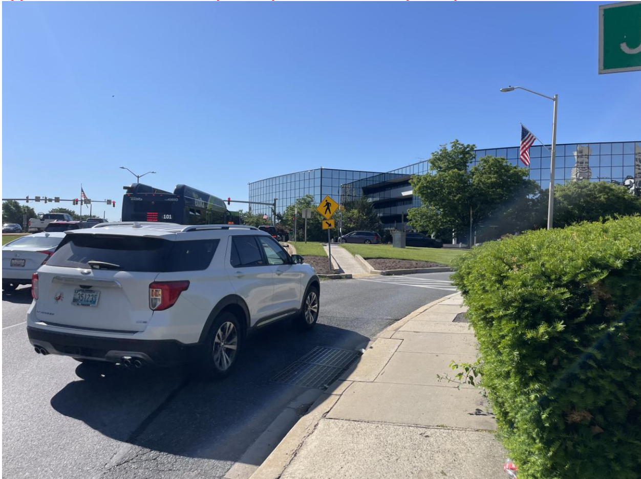
Figure 137. Faded pedestrian crosswalks along the eastbound, westbound, and southbound (show below) approach slip lanes with poor visibility of crosswalks from approach #21 - Rockville Pike (MD 355) & Veirs Mill Road (MD 28)
