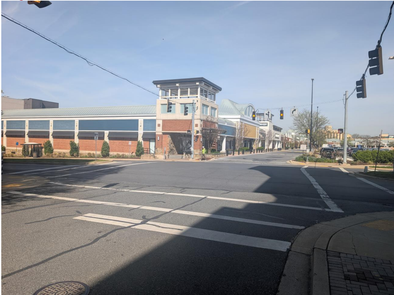
Figure 53. Existing crosswalks at all approaches of Intersection #8 - Halpine Road and Congressional Plaza
