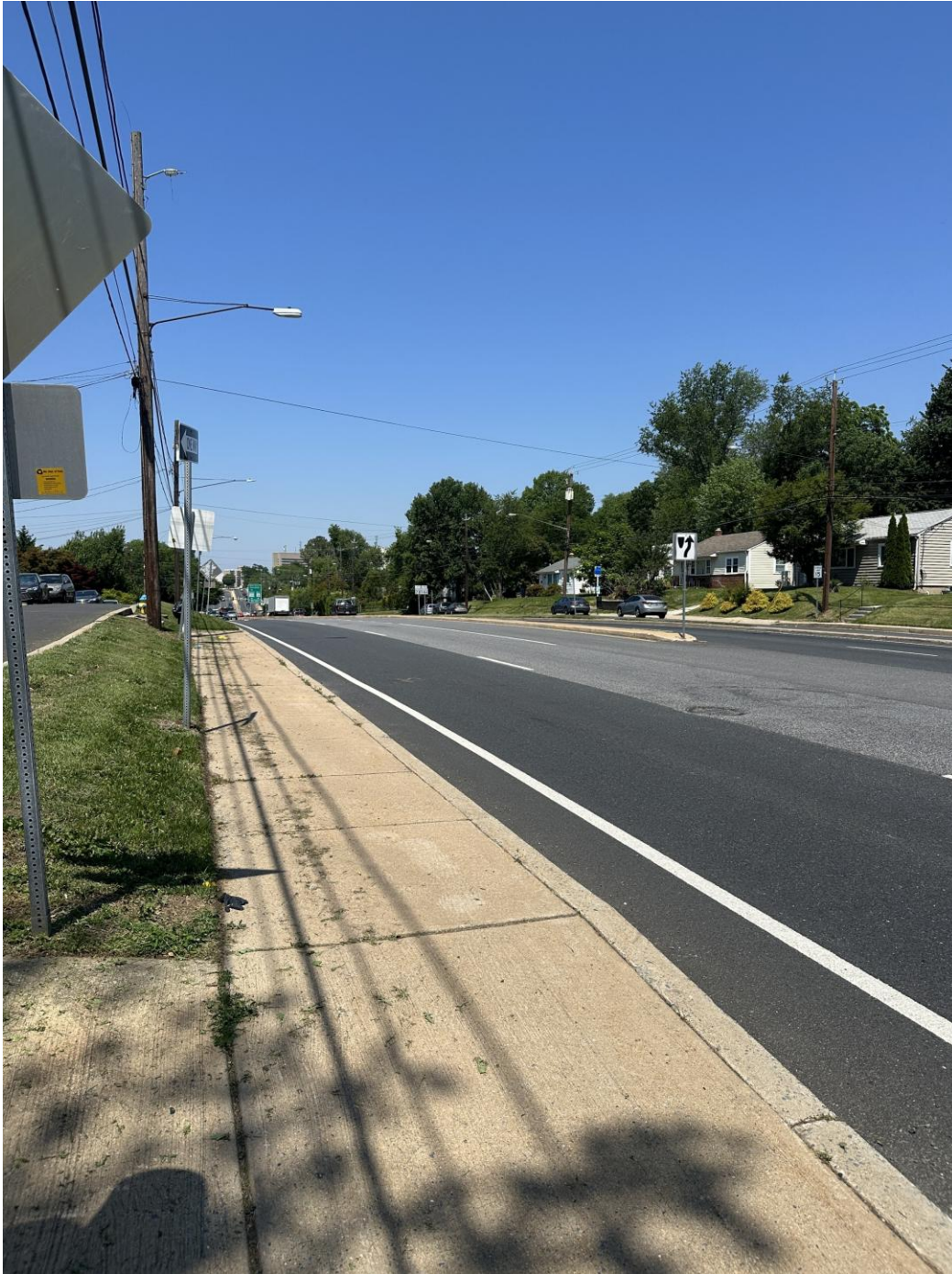
Figure 187. Uncontrolled crosswalk near the crest of a hill at Intersection #29 - Veirs Mill Road (MD 586) & Woodburn Road
