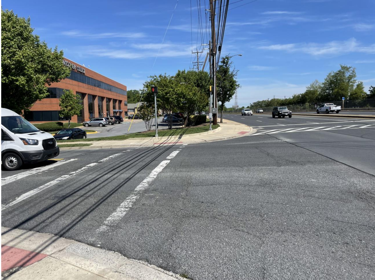
Figure 92. Pedestrian crosswalk on the west leg with deteriorated pavement marking lacking a high-visibility pattern #14 - Hungerford Drive (MD 355) & Mannakee Street
