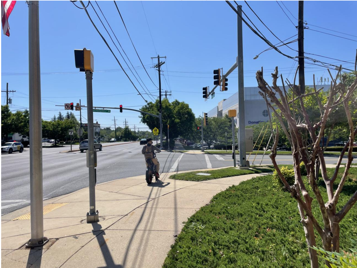
Figure 152. Pedestrian crosswalks on the east and west legs lack a high-visibility design #23 - Rockville Pike (MD 355) & Richard Montgomery Street
