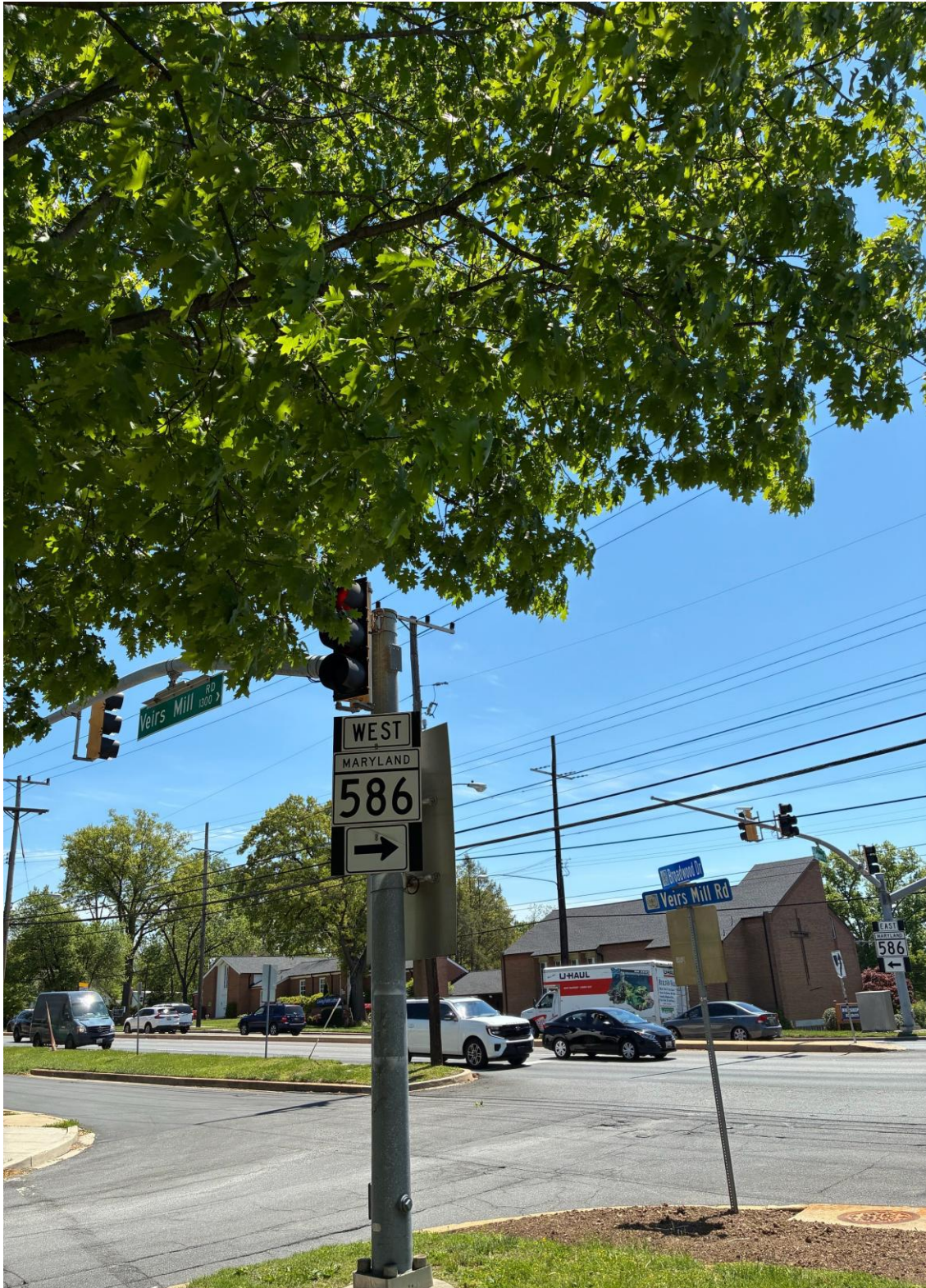
Figure 100. Obstructed signal head at Intersection #15 - Veirs Mill Road (MD 586) & Broadwood Drive
