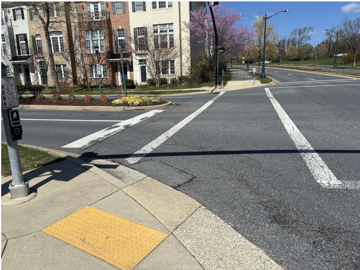
Figure 41. Wide curb radii allow drivers to turn right at high speeds off of Gaither Road at Intersection #6 – Gaither Road & Piccard Drive
