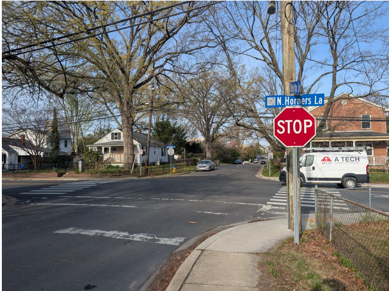
Figure 66. Faded stop bar and crosswalk markings at westbound Baltimore Road at Intersection #10 – Woodland Road & N. Horners Lane
