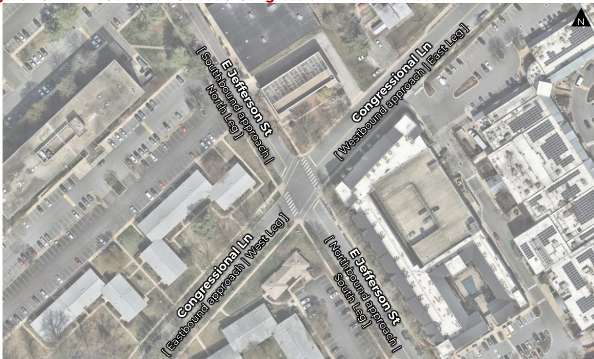
Figure 45. #7 – E. Jefferson Street & Congressional Lane Intersection
