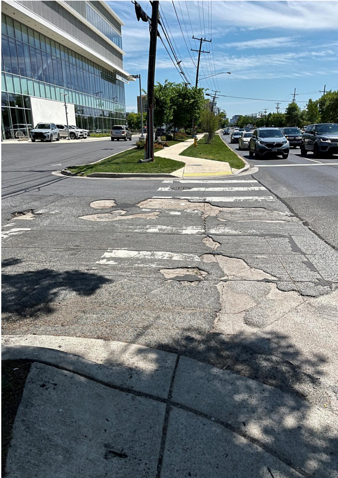
Figure 113. Missing pedestrian signal heads on the westbound approach at Intersection #17 - Rockville Pike (MD 355) & Templeton Place
