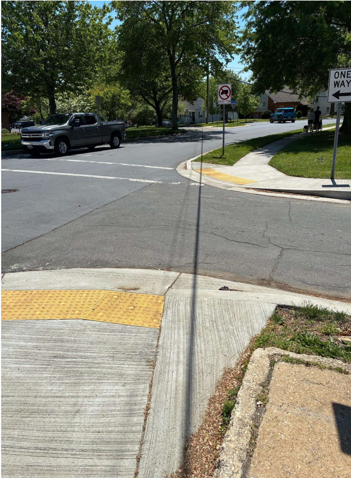
Figure 101. Missing crosswalk on frontage road at Intersection #15 - Veirs Mill Road (MD 586) & Broadwood Drive
