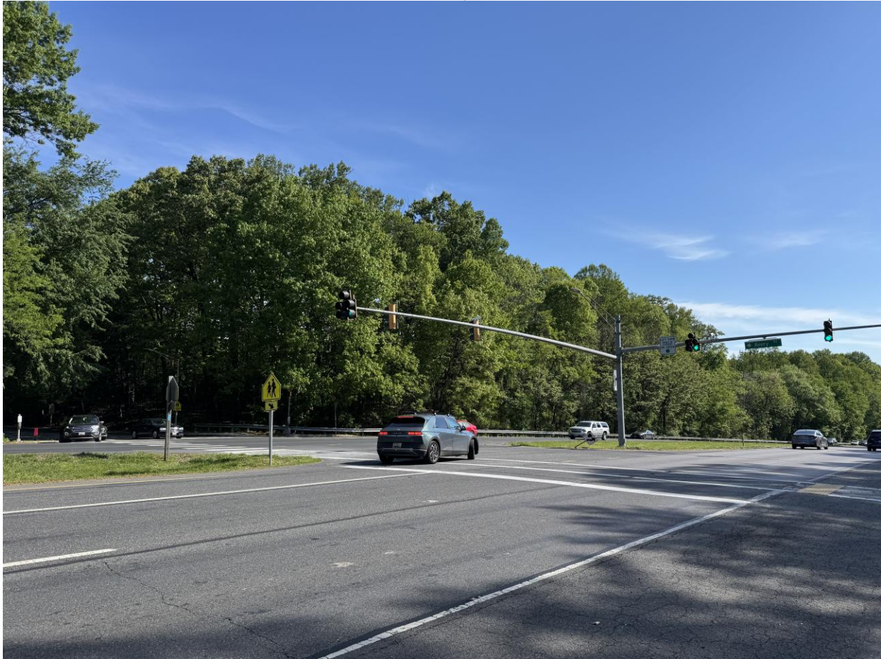
Figure 119. Vehicles turning on a permissive left turn from eastbound Norbeck to northbound Avery. Three head on left turn crashes and 138 near misses occurred in this movement. #18 - Norbeck Road (MD 28) & Avery Road
