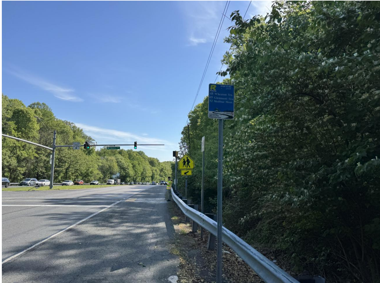
Figure 120. Lack of separated pedestrian facility on the south leg of eastbound approach between crosswalk and bus stop #18 - Norbeck Road (MD 28) & Avery Road
