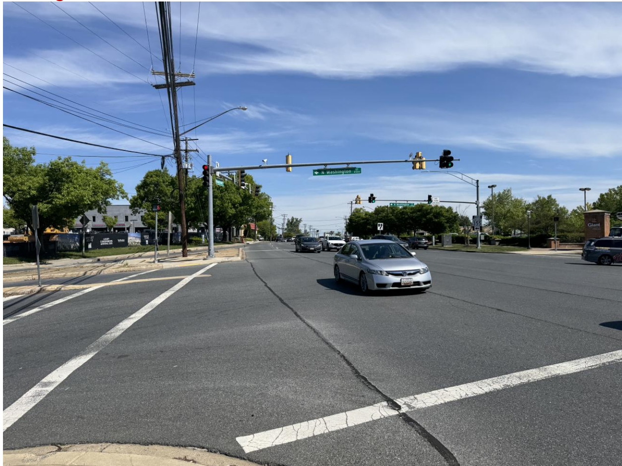
Figure 80. Lack of puppy tracks in intersection, particularly for eastbound left-turn movement, with frequent RideOn bus traffic #12 - Hungerford Drive (MD 355) & N. Washington Street
