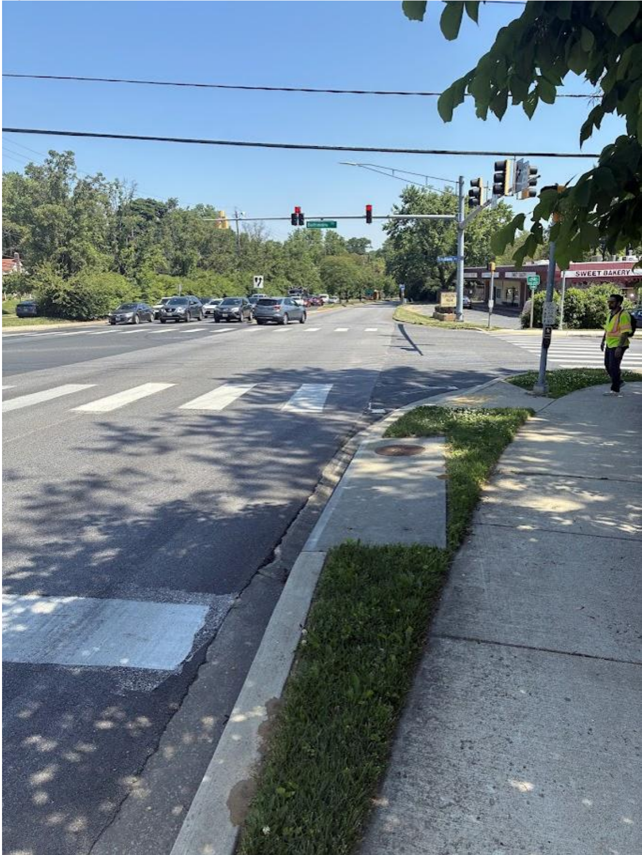
Figure 145. Wide curb radius at Intersection #22 - First Street (MD 28) & Baltimore Road
