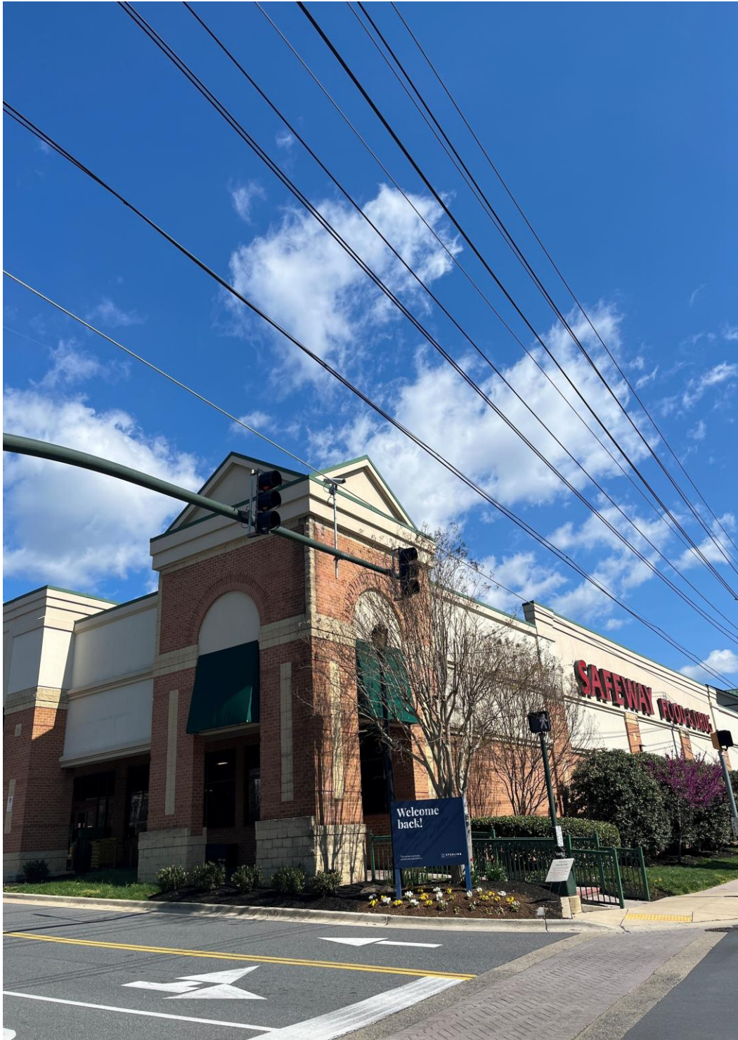
Figure 37. Lack of ADA-Compliant access on the northwest corner at Intersection #5 – Redland Boulevard & Thompson Dairy Way
