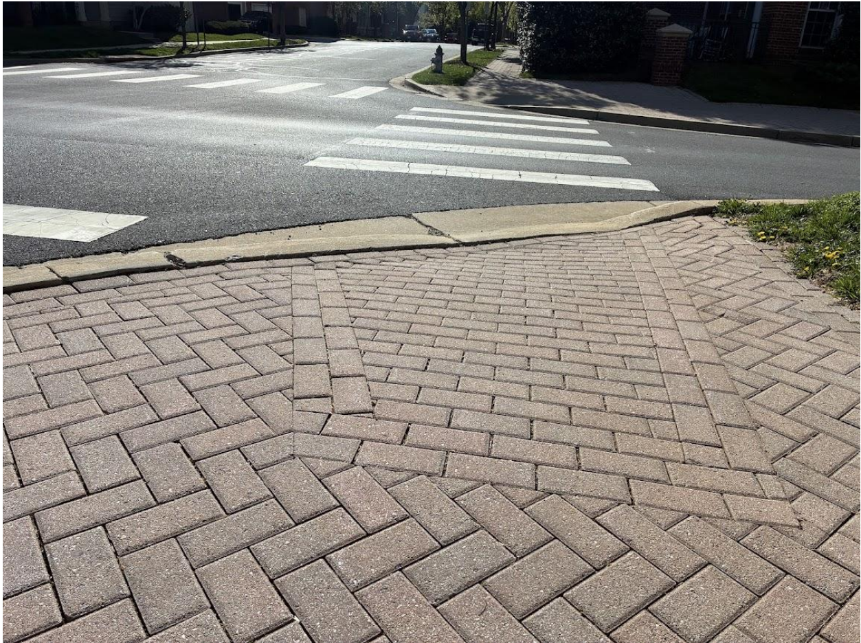
Figure 23: Median sidewalk at Intersection #3 – King Farm Boulevard & Grand Champion Drive
