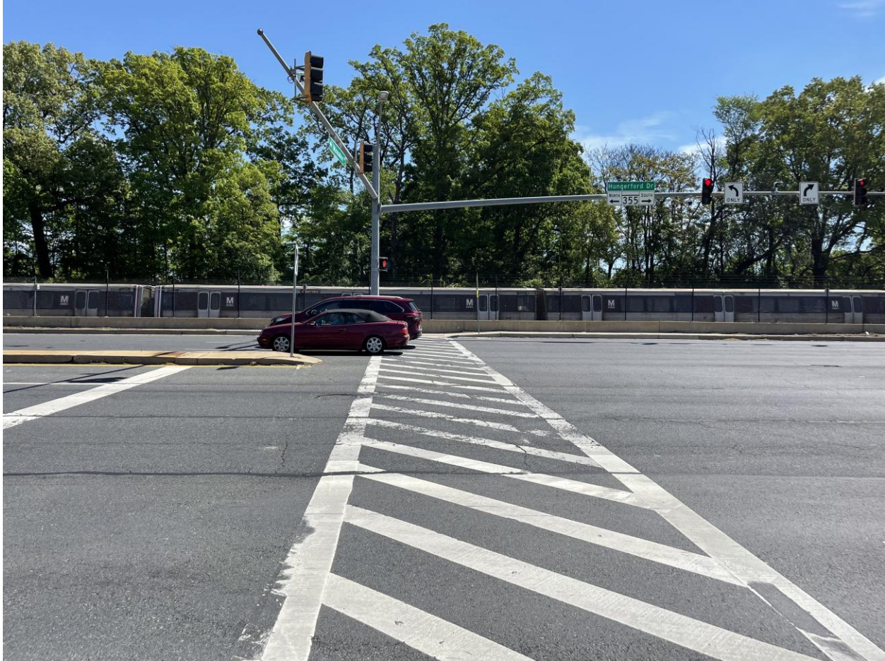
Figure 93. Long pedestrian crosswalk on north leg with deteriorated pavement marking #14 - Hungerford Drive (MD 355) & Mannakee Street
