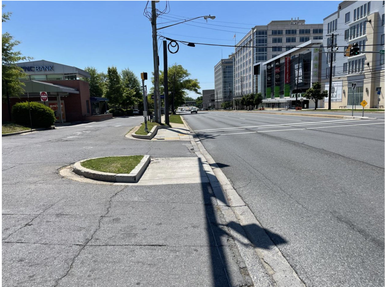
Figure 165. Unmarked pedestrian crosswalk over driveways on east leg #25 - Hungerford Drive (MD 355) & Beall Avenue
