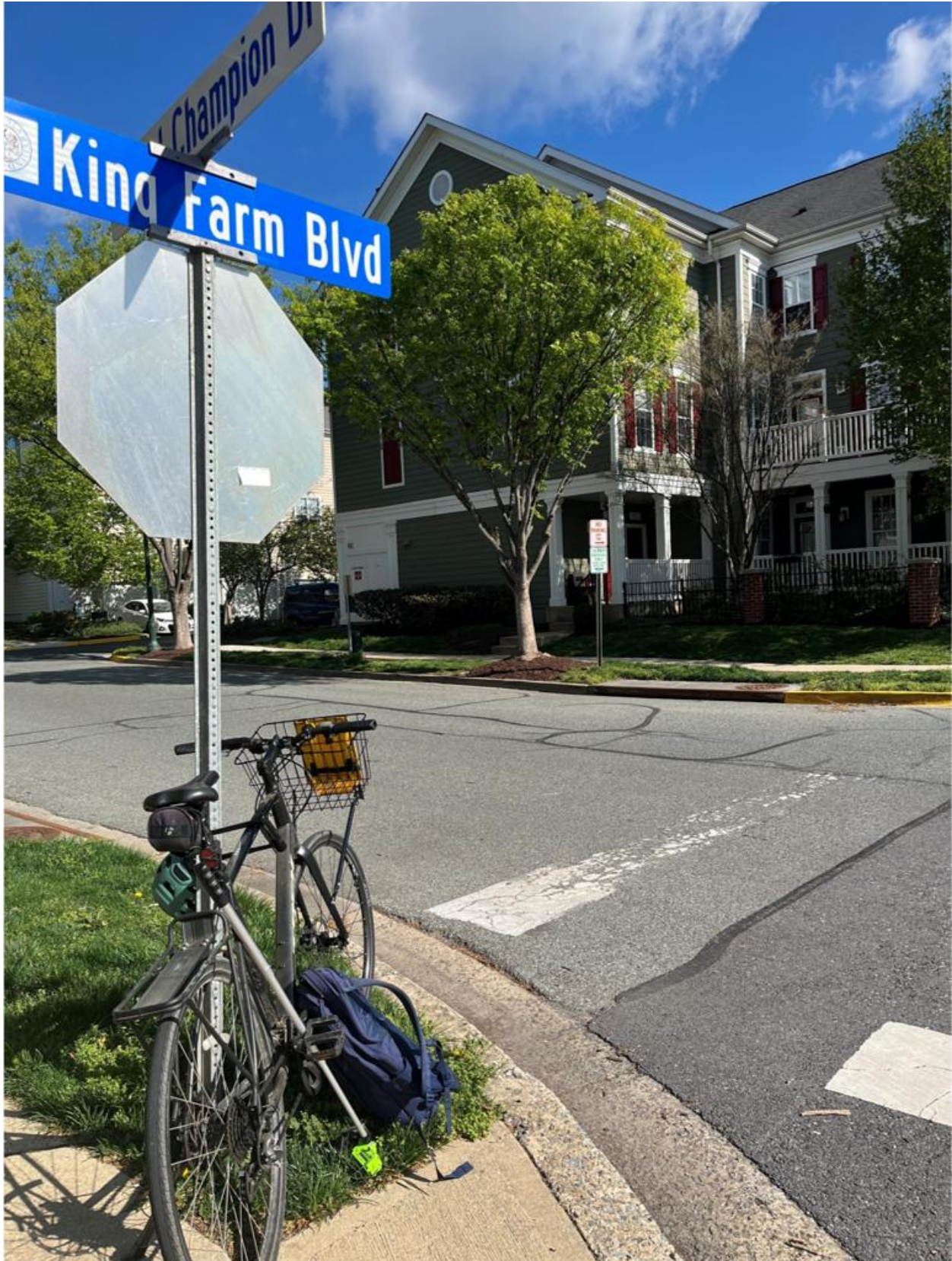
Figure 24: West leg faded stop bar at Intersection #3 – King Farm Boulevard & Grand Champion Drive
